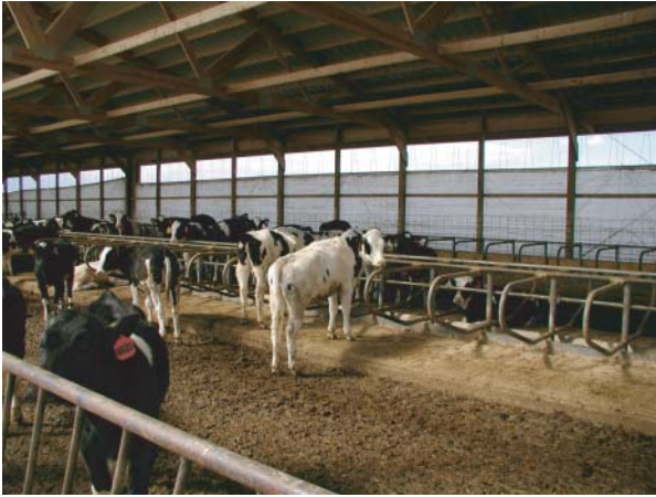
Figure 34.6 Monopitch building for young stock, with curtain sides that can be raised or lowered to improve ventilation, depending on the weather.
