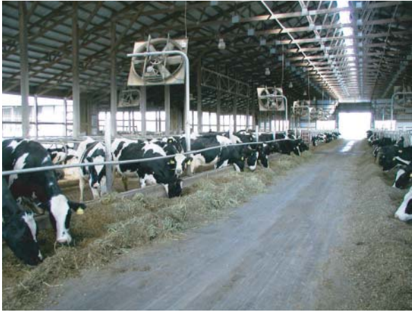
Figure 34.3 A well-designed building used to house dairy cattle all year round. Good ventilation from open sides and the option to increase cooling in hot weather.
