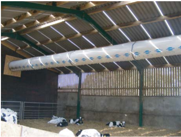
Figure 34.4 Forced air systems such as this can hugely improve ventilation especially for young stock.
