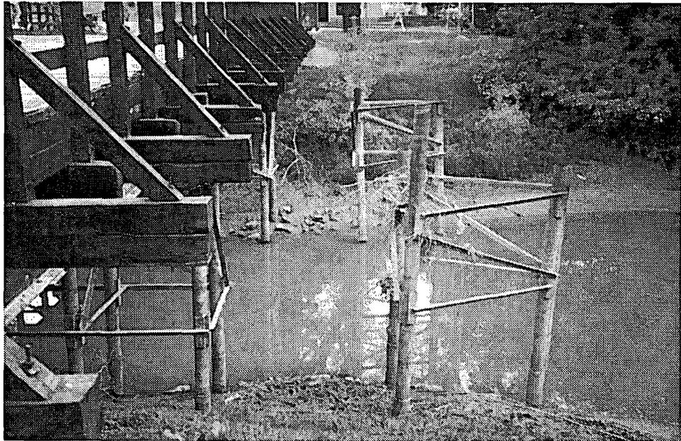
**Figure 5.14** *Sacrificial piles upstream of a bridge*
