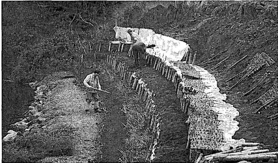
**Figure 5.28** Construction of rock armour and willow faggoting repair to eroded river bank
