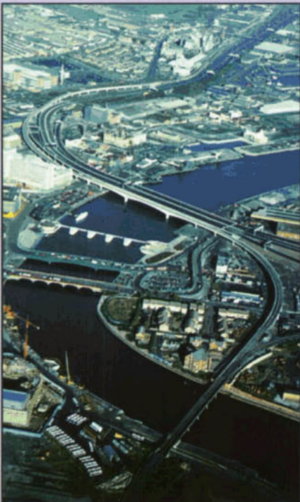
Below right: Figure 34 Construction of Cross Harbour Link
