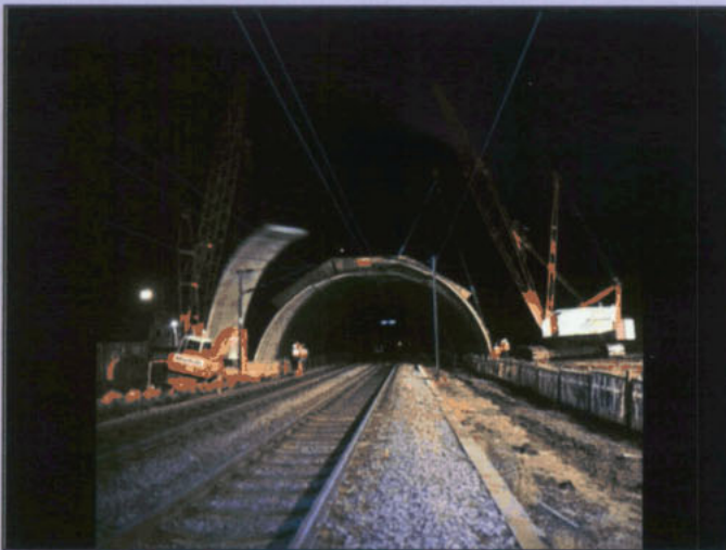
Below right: Figure 28 Overview of New Cowdens Railway Bridge
