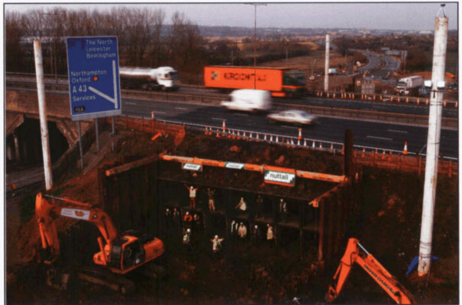
Figure 17 Concrete box jacked under the M1
