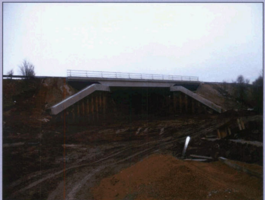
Figure 18 Construction of Top Lane Underpass
