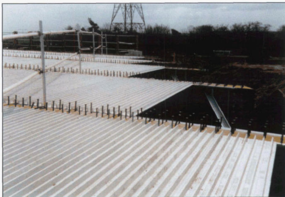
Figure 4 GRP panels used with steel beams
