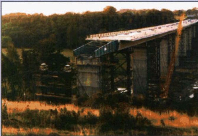
Below right: Figure 38 Overview of Ceiriog Viaduct
