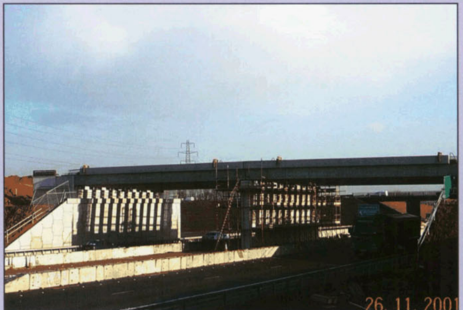
Figure 23 Construction of new overbridge
