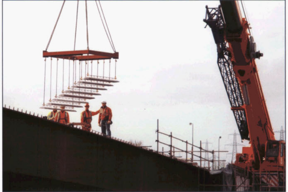
Figure 2 Purpose-made lifting frame for lattice girder units
