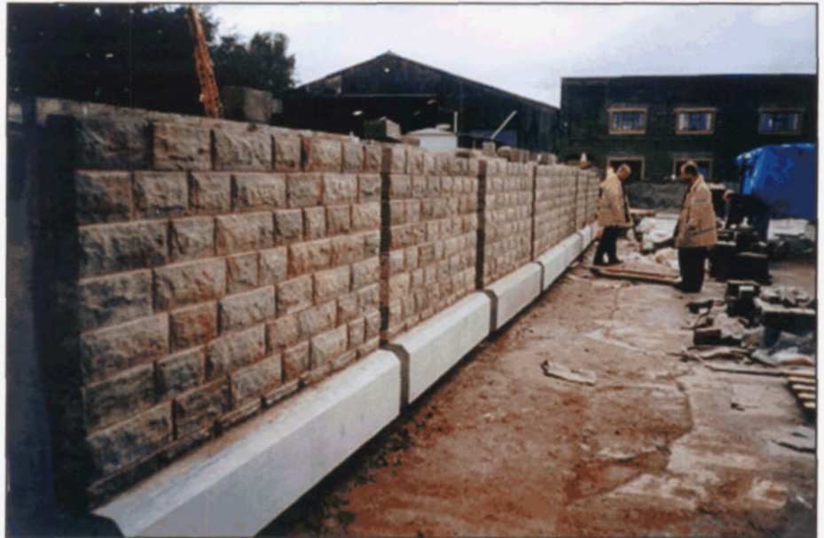
Figure 15 Parapet clad with masonry
