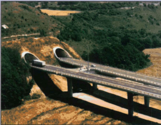
Below right: Figure 32 Construction of Roundhill Viaduct
