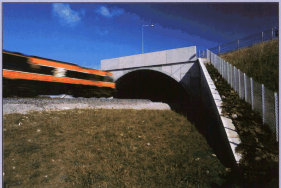
Figure 26 Lagavooren Bridge over railway
