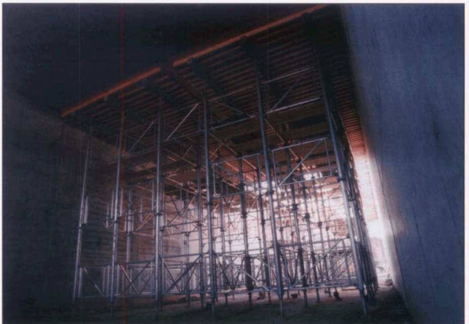
Figure 10 Traveller being used for construction of soffit of underpass
