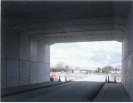
Figure 12 Underpass formed from open cell units
