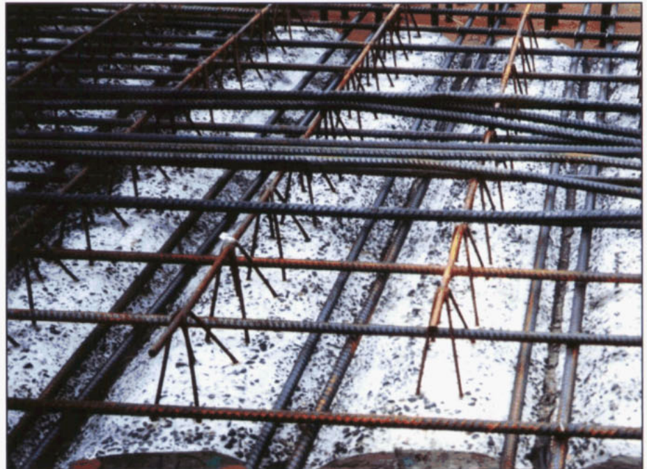
Figure 3 Lattice girder units in place
