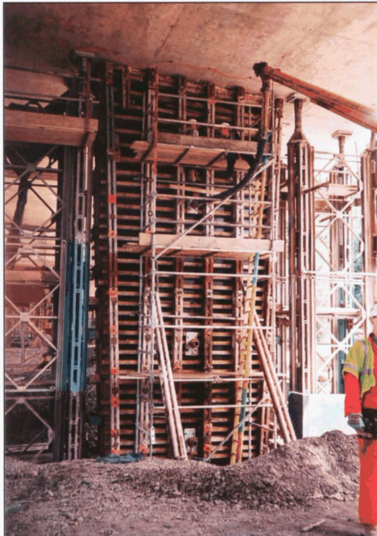
Figure 7 Self-compacting concrete being used for the reconstruction of a bridge pier
