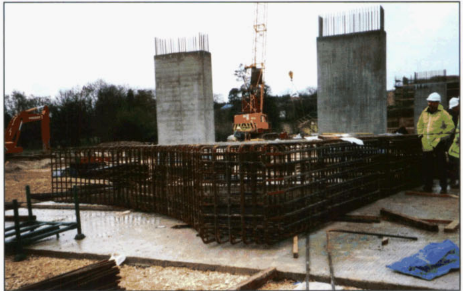
Figure 8 Prefabricated reinforcement for pier crosshead
