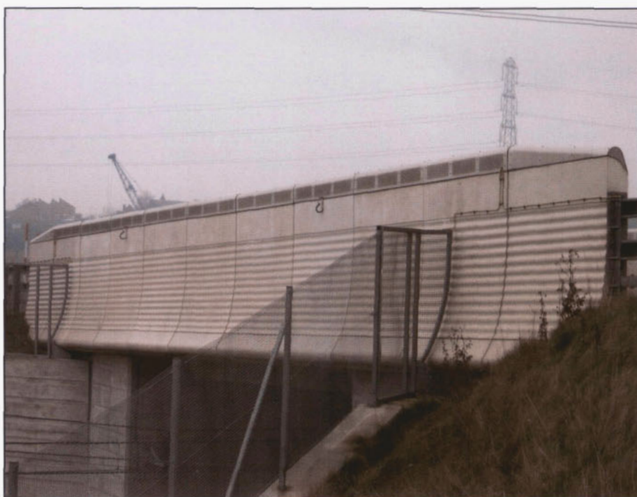
Figure 1 Parapet on Channel Tunnel Rail Link
