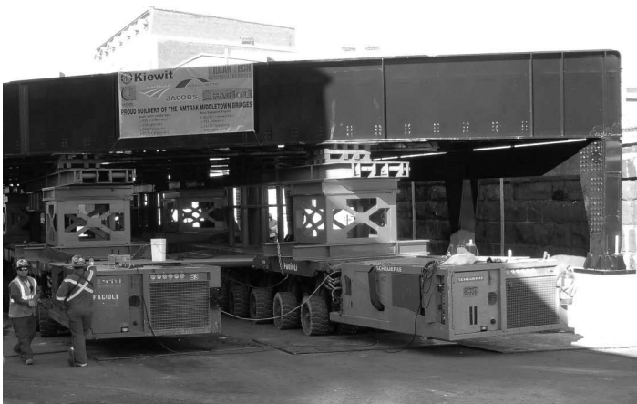
FIGURE 11.23 Span erection with SPMT. (Courtesy J. Richter. © Amtrak, Philadelphia, PA, USA.)
