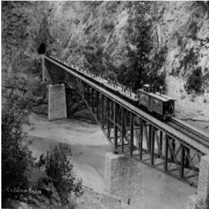
FIGURE 1.16 Fraser River Bridge built in 1884, British Columbia, Canada. (Photo by J. A. Brock, Canadian Pacific Archives NS.11416.)
