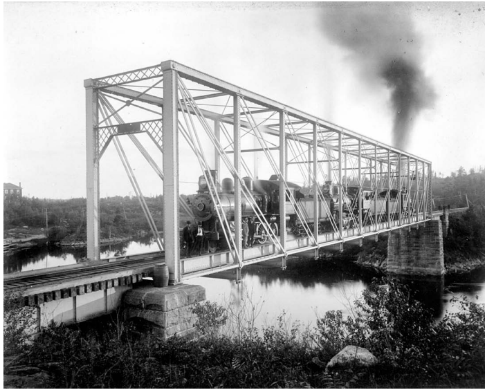
FIGURE 1.3 Whipple truss span. (Courtesy of the author, Canadian Pacific Engineering.)
