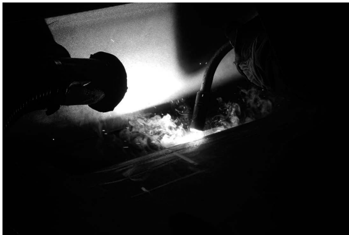
FIGURE 10.18 FCAW welding. (Courtesy of Y. Martin, Canam Bridges Inc., St. Foy, QC, Canada. With permission.)
