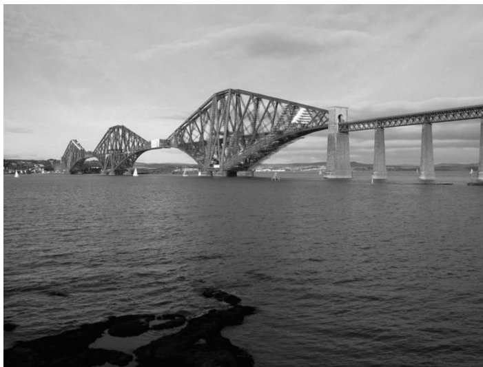
FIGURE 1.17 The Forth Rail Bridge built over the Firth of Forth in 1890, Scotland. (From GFDL Andrew Bell, http://en.wikipedia , January 2005.)
