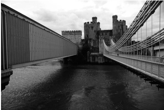
FIGURE 1.5 The Conwy Bridges: Stephenson's Tubular Railway Bridge built in 1848 and Thomas Telford's Suspension Highway Bridge built in 1826 at Conwy Castle, Wales. (From Stephen J. Hill, Redwood City, CA. With permission.)
