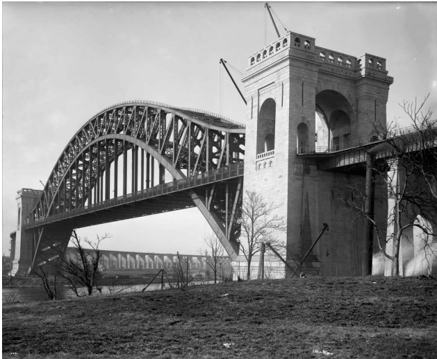
FIGURE 1.20 The Hell Gate Bridge built across the East River in 1916, New York. (Courtesy of Library of Congress from Detroit Publishing Co.)
