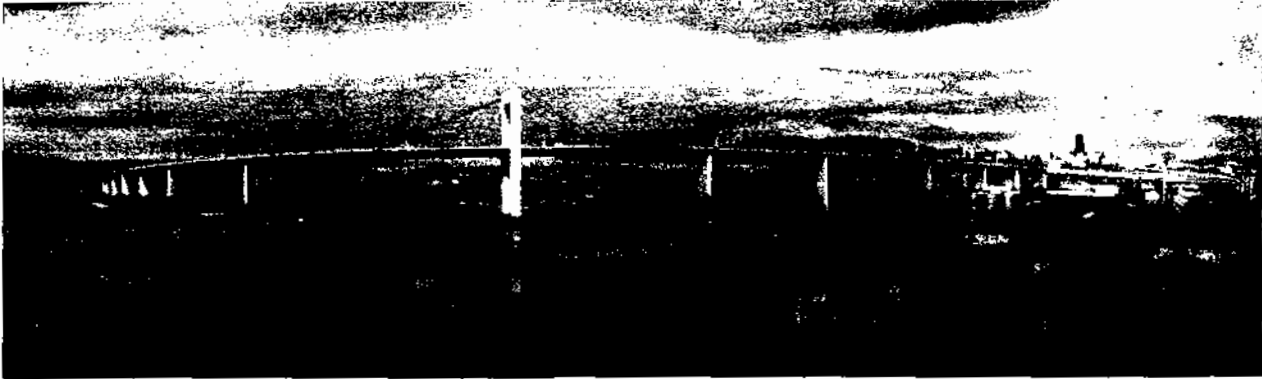
FIGURE 1.26 West Seattle freeway bridge. (Courtesy of J. E. Arnberg, City of Seattle Department of Engineering.)
