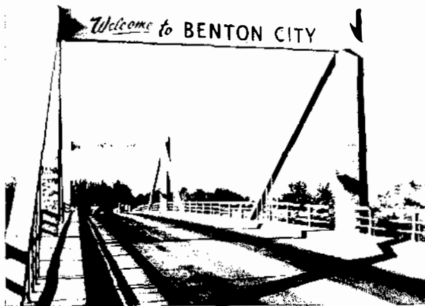
FIGURE 1.20 Benton City Bridge, Washington. (Courtesy of John H. Garren, FHWA Washington Division.)
