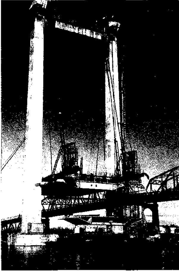
FIGURE 4.26 Pasco-Kennewick Intercity Bridge, erection of precast segments from barge. (Courtesy of Arvid Grant.)
