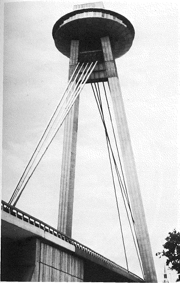
FIGURE 5.34 Bratislava Bridge, tower showing stay arrangement. (Courtesy of John H. Garren, FHWA Region 10.)
