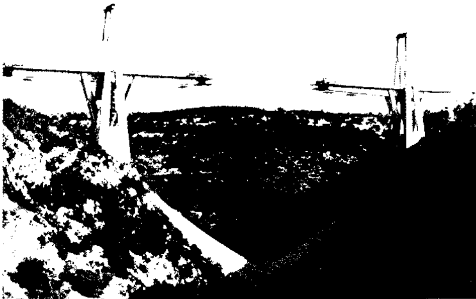
FIGURE 4.4 Wadi Kuf Bridge, general construction view. (Courtesy of R. Morandi.)
