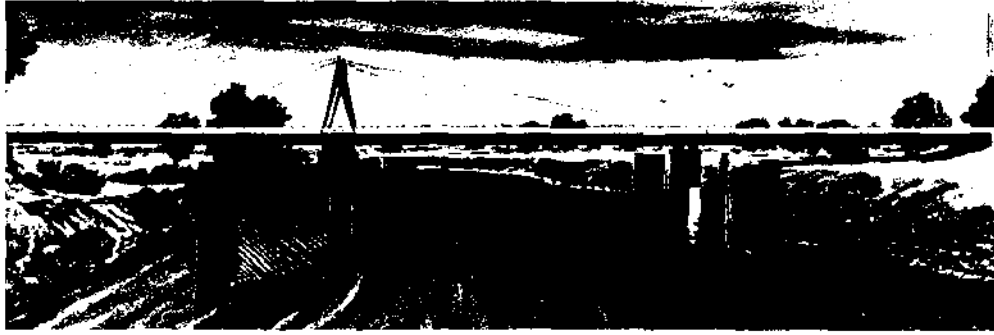
FIGURE 1.29 Cable-stay swing span; Meridian, California. (Courtesy Department of Transportation, Division of Highways, Office of Structures, State of California.)
