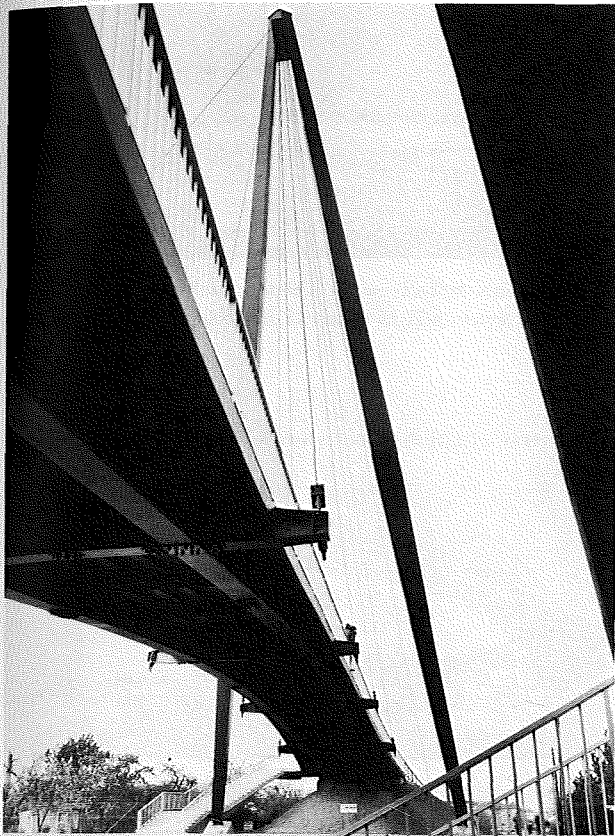
FIGURE 7.17 Raxstrasse Footbridge. (Courtesy of Waagner-Biro Aktiengesellschaft, Vienna.)
