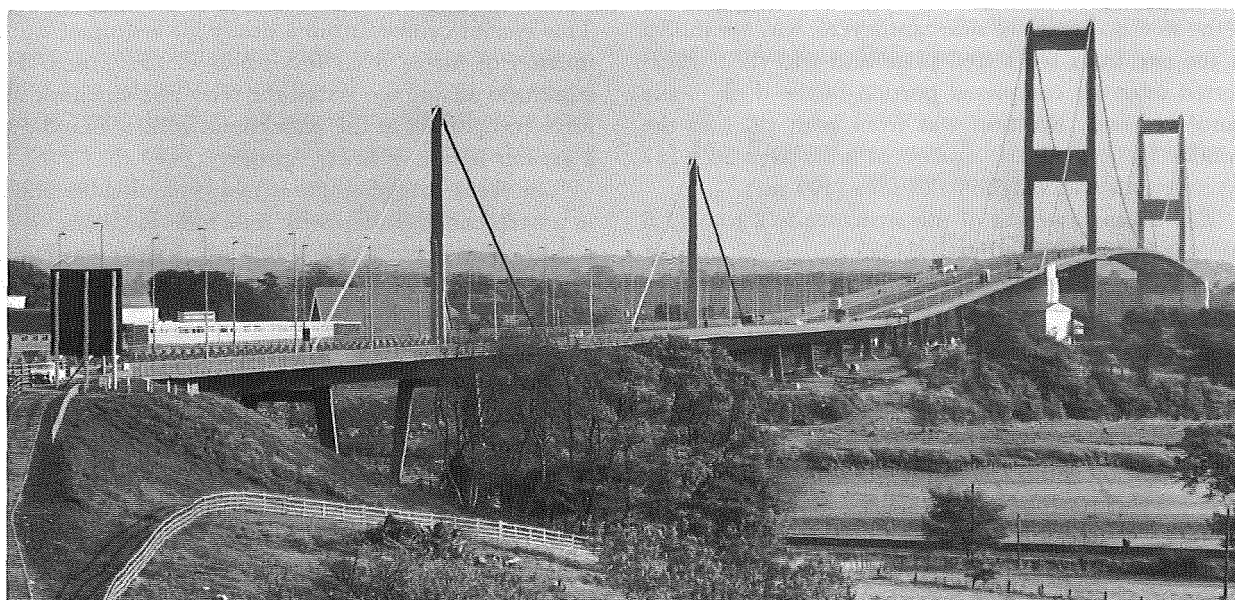
FIGURE 5.12 Wye Bridge, Severn Bridge in background. (Courtesy of The British Constructional Steelwork Association, Ltd.)
