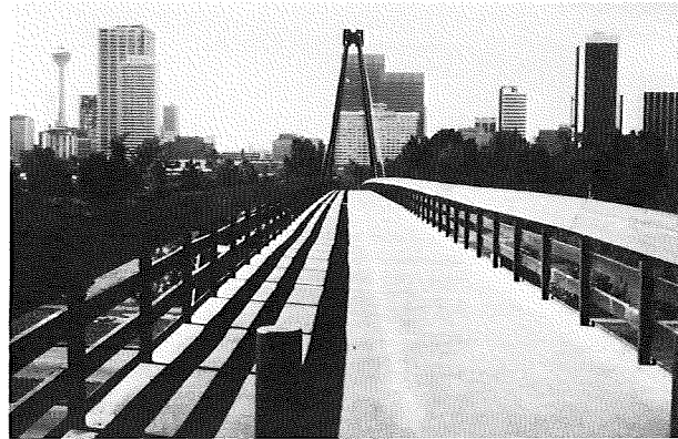
FIGURE 7.26 Prince's Island Pedestrian Bridge, longitudinal view of deck. (Courtesy of Joseph A. Chilstrom, FHWA, Washington Division.)
