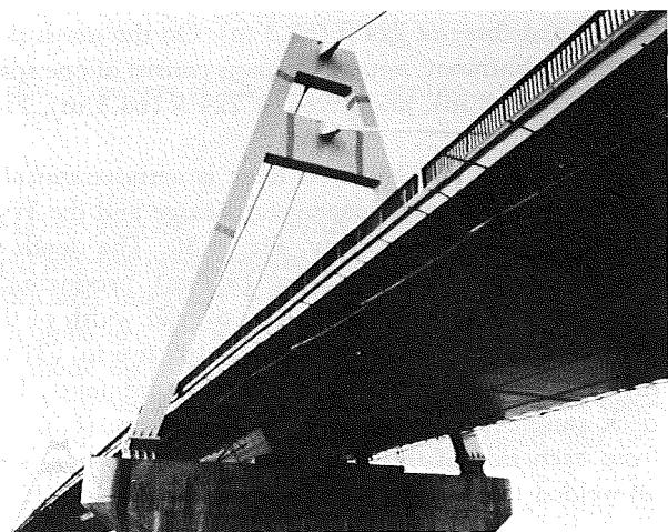
FIGURE 5.27 Toyosato-Ohhashi Bridge, Osaka, Japan.
