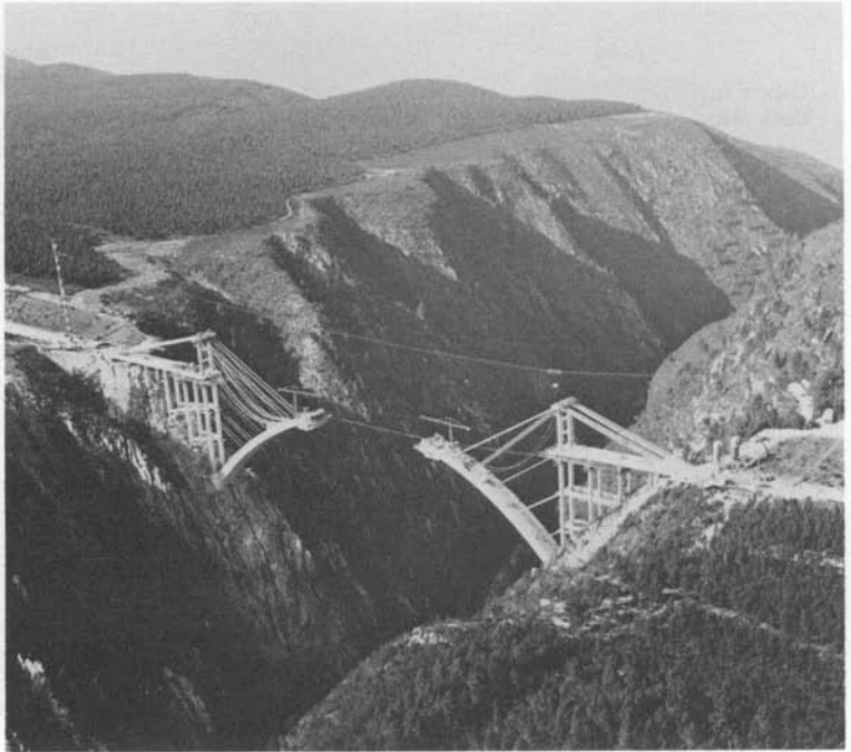
Figure 5.10 Bloukrans Bridge, South Africa
