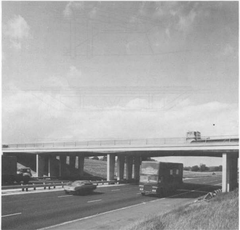
Figure 1.30 Motorway bridge in England (courtesy of Freeman, Fox and Partners)
