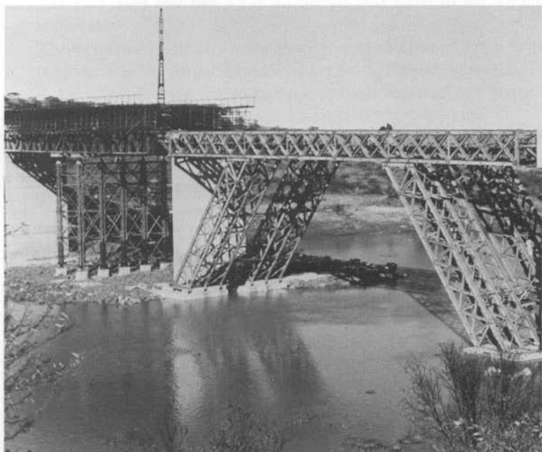
Figure 5.2 Bridge over the Vaal River, South Africa
