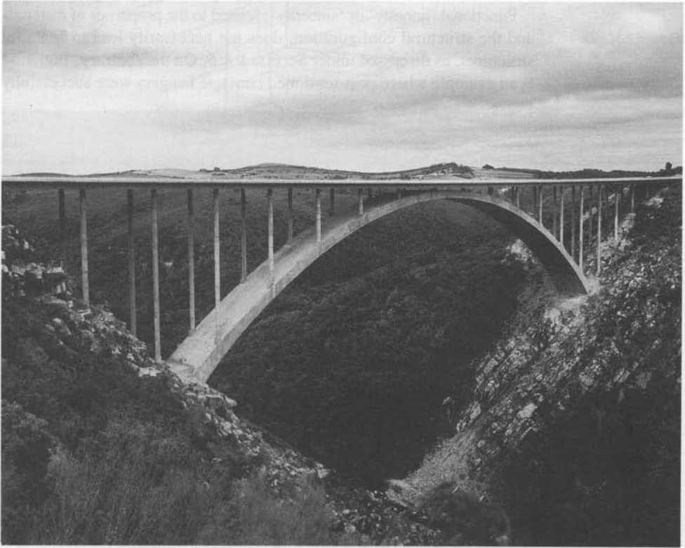
Figure 1.33 Bridge over Van Staden's Gorge in South Africa
