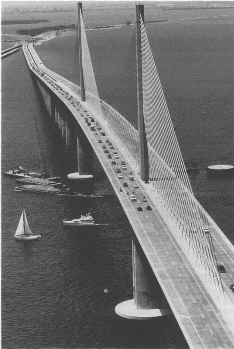
Figure 5.49 Sunshine Skyway Bridge, Florida, USA (courtesy of Dr P Marti, VSL International)
