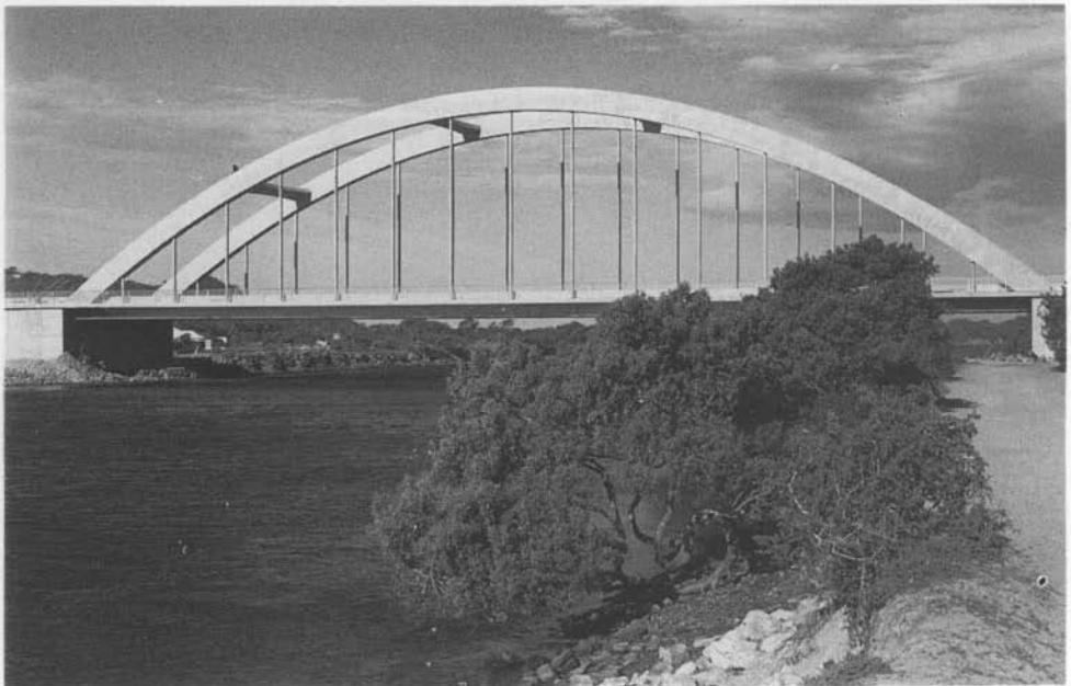
Figure 1.34 Tied arch bridge at Port Alfred, South Africa
