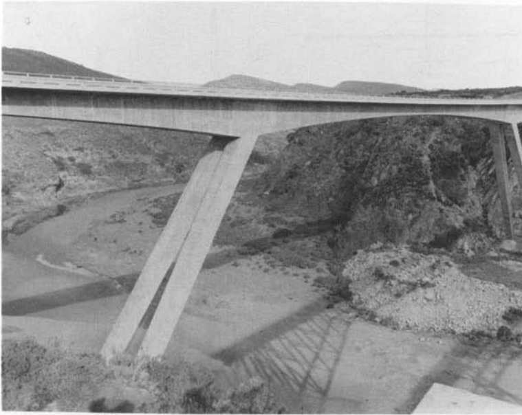
Figure 1.20 Strut-frame over Gouritz River, South Africa
