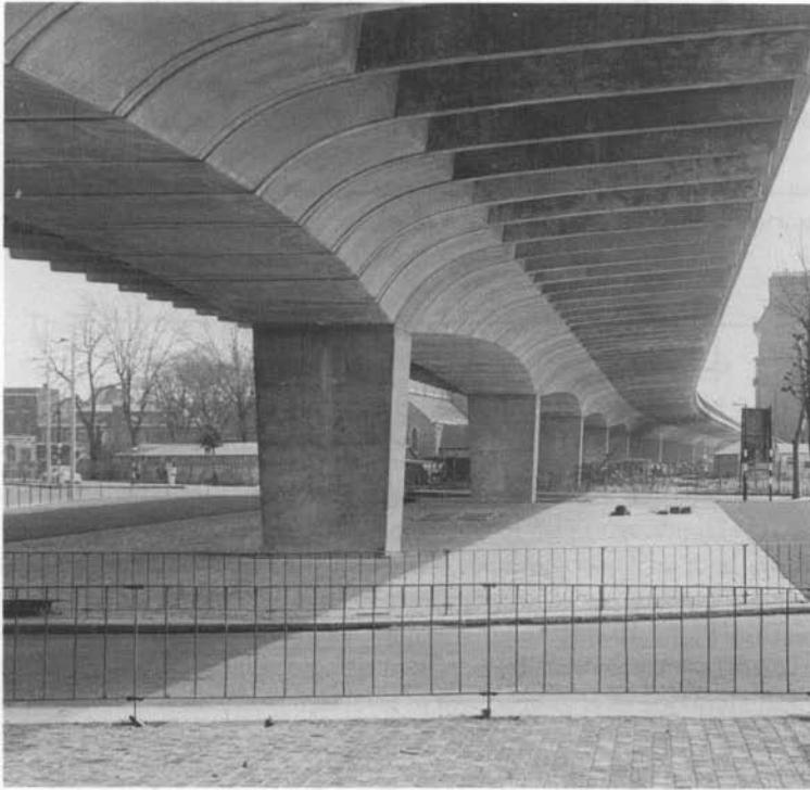
Figure 5.34 Hammersmith Flyover, London (courtesy of Maunsell and Partners)
