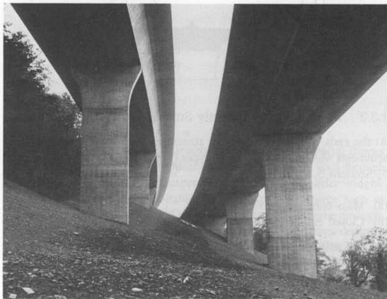
Figure 1.18 Wynhol Viaduct, Clevedon Hills, England (courtesy of Freeman, Fox and Partners)
