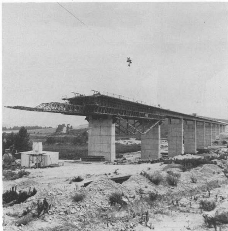
Figure 5.4 Draaiberg Bridge near Cape Town, South Africa (courtesy of R. Meuwese)
