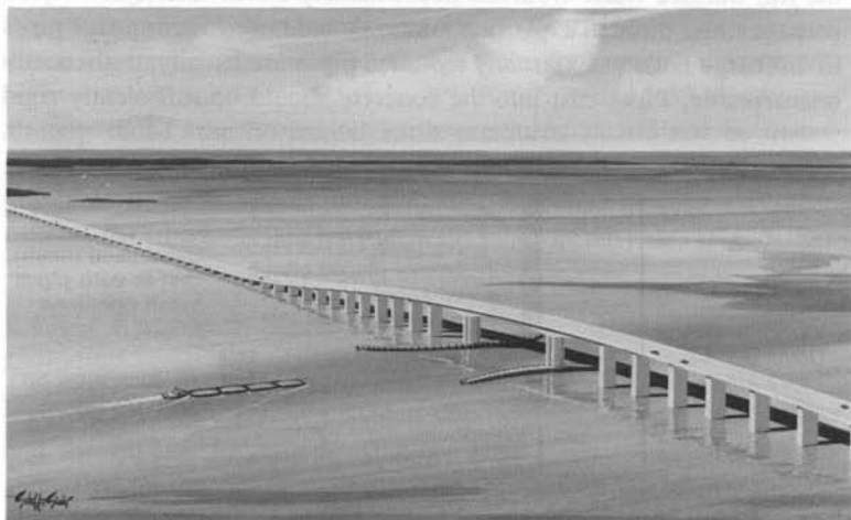
Figure 5.21 Dauphin Island Bridge (courtesy of Figg and Muller Engineers Inc)
