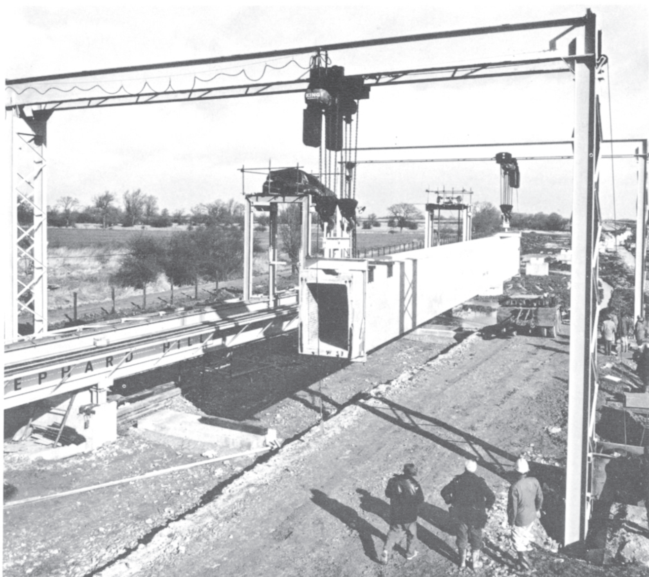
Figure 15. Erecting beam for hovercraft track.
