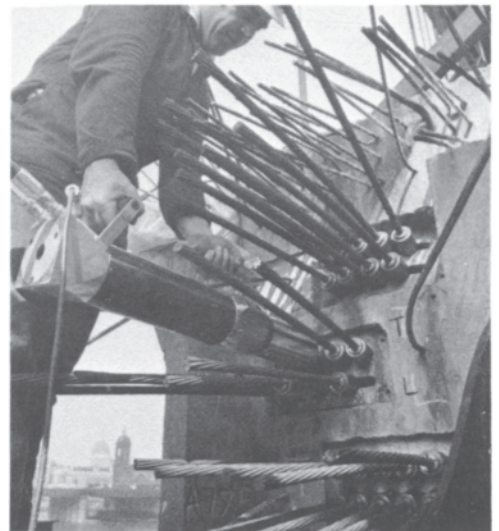
Below: Individual stressing of strands in a cable.
