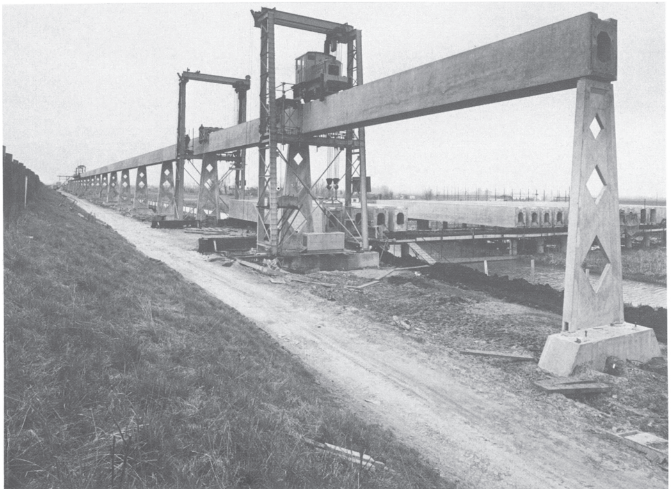
Figure 14. Precast concrete track for experimental tracked hovercraft.
