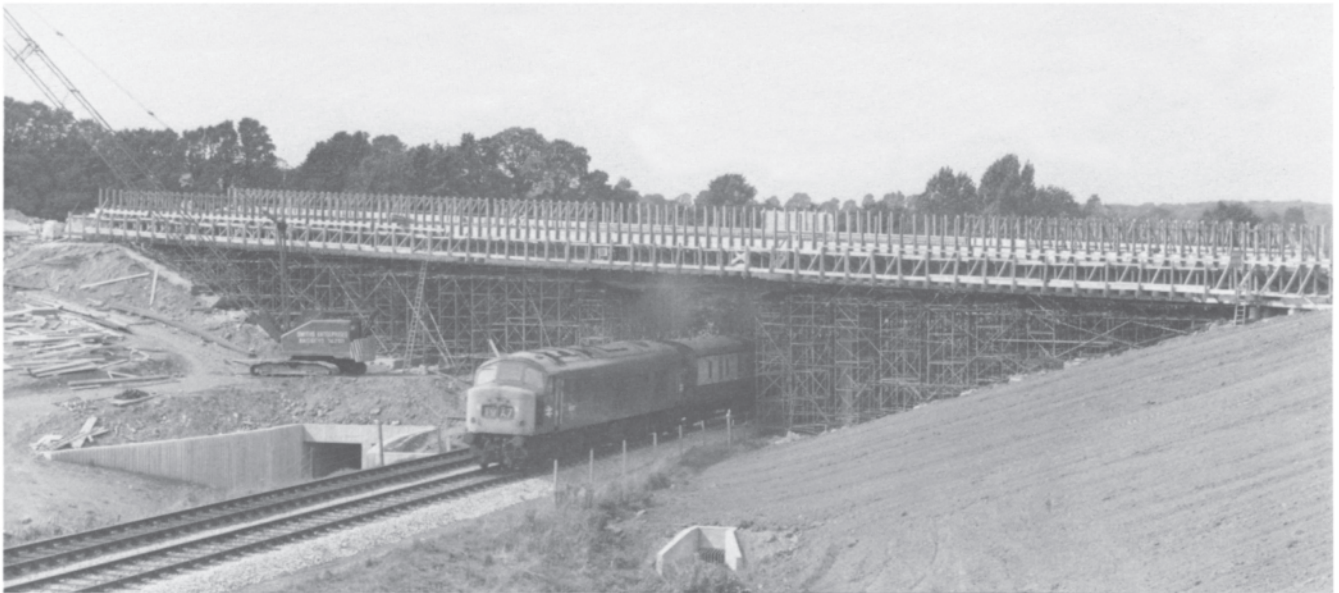
Figure 25. Falsework for bridge deck.
