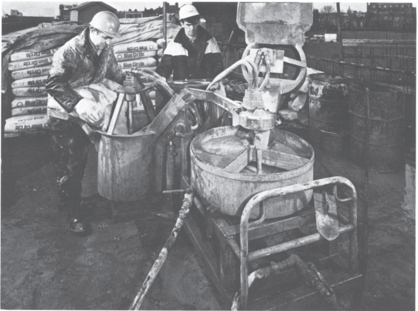
Figure 10. Equipment for grouting prestressing cable ducts under pressure. High-speed mixer and storage bin with continuous agitation.
