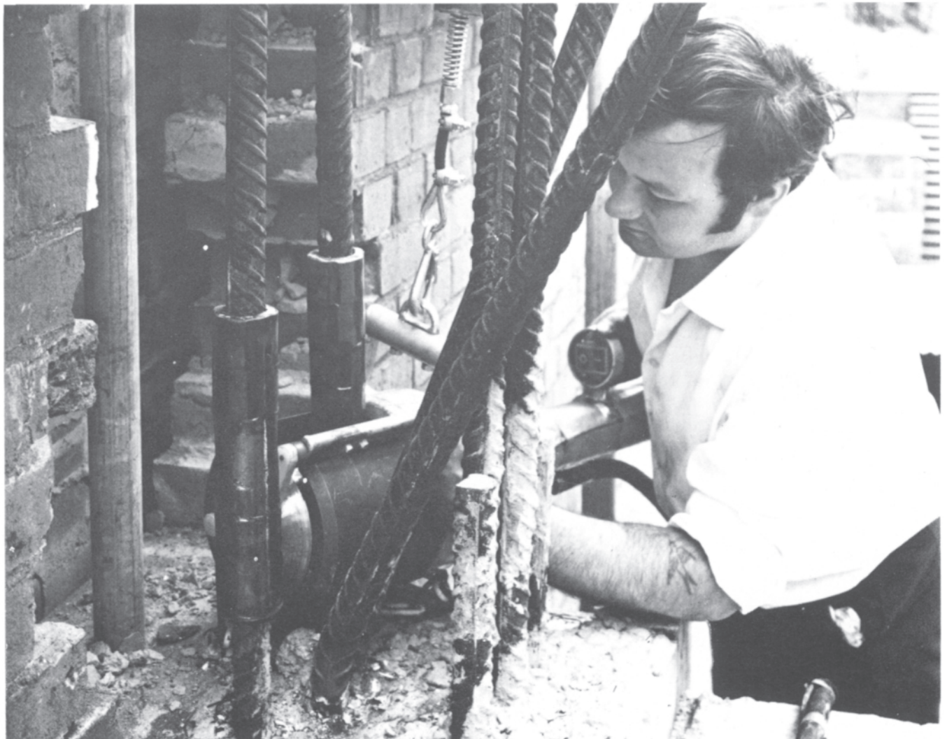
Figure 9. Mechanical splicing of reinforcement by swaging.
