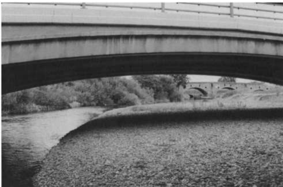
Fig. 4.27 The problem of three bridges in close proximity causing hydraulic interference. The most modern upstream bridge has a large single span, through which can be seen a four-span masonry arch bridge, through which can be seen the low spans of a brick bridge carrying the Trent and Mersey Canal over the River Dove. The openings of the latter regularly submerge during flood.
