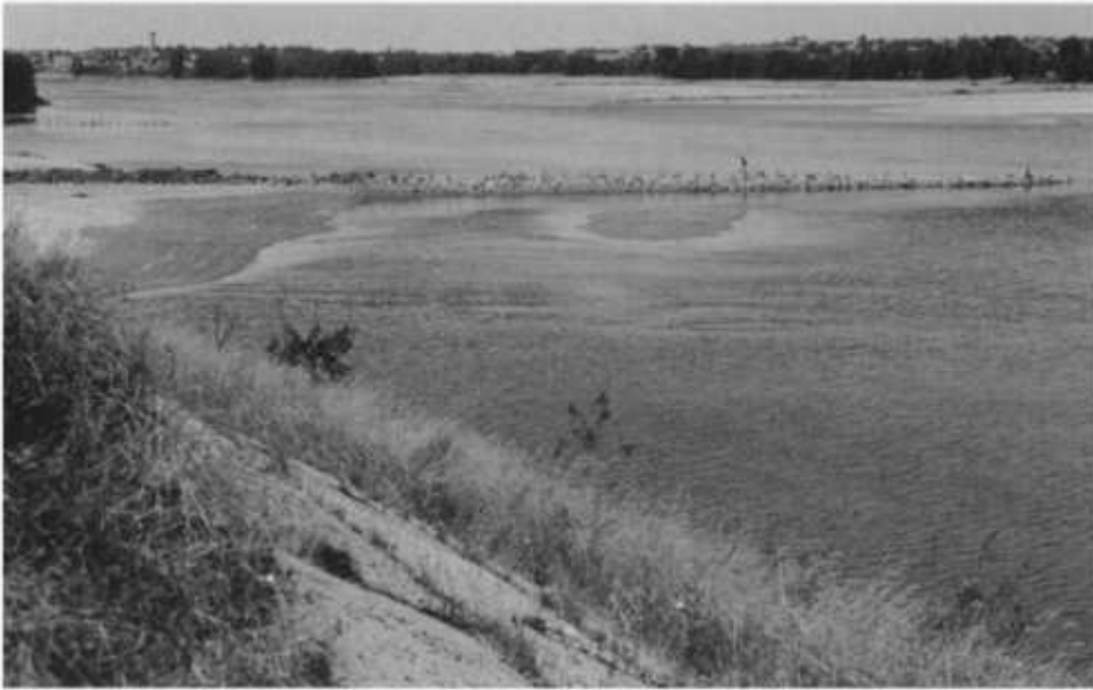
Fig. 7.19 Groynes on the River Loire, France, with a concrete revetment on the bank. The flow is away from the camera. Note the size (the people on the groyne are barely visible) and the siltation, especially on the opposite bank.
