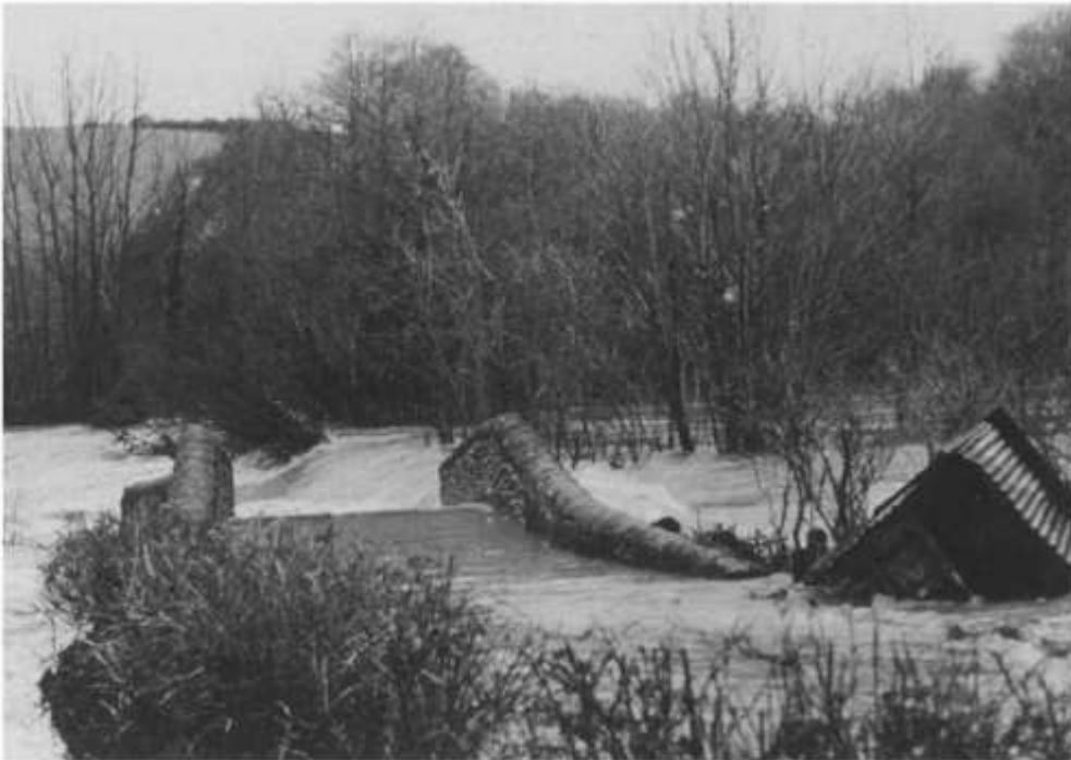
Fig. 6.1 Floodwater passing from right to left over the bridge approach at Chilly Bridge on the River Exe, December 1960. Preventing this flow by raising the approach embankments would increase the chance of the bridge being damaged and exacerbate flooding upstream. The object at the bottom right is reputedly a garden shed, which illustrates the hazard of debris becoming trapped in an opening. (Reproduced by permission of the Environment Agency)
