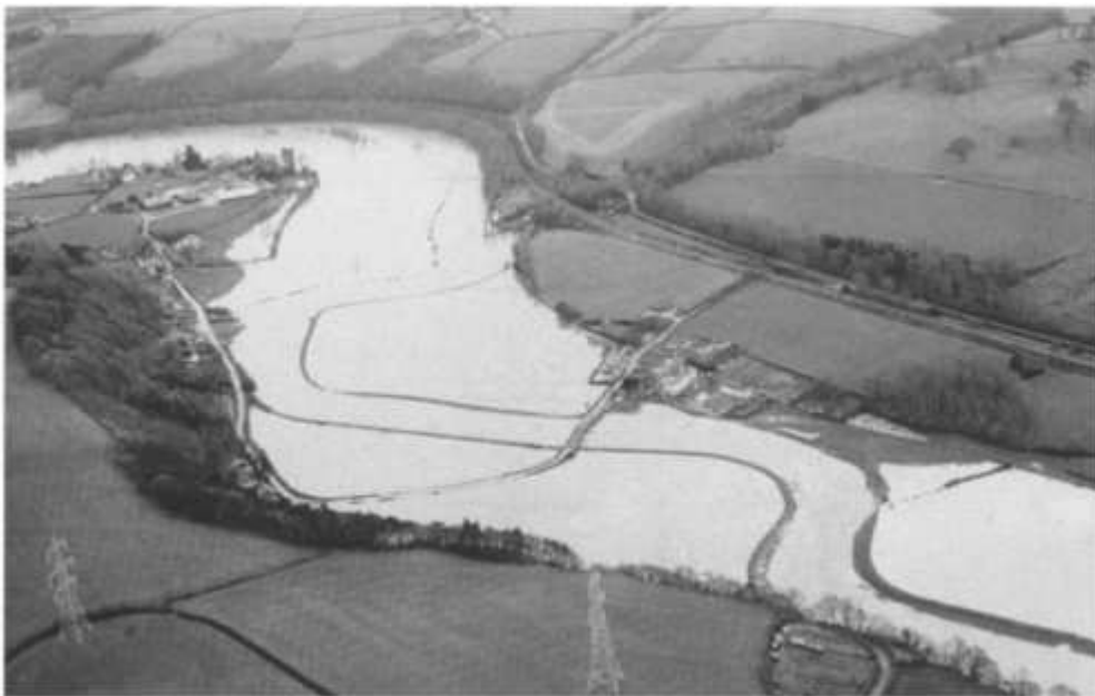
Fig. 8.16 Halfpenny Bridge on the River Torridge at Weare Gifford, December 1979. The presence of levees poses some questions with respect to the hydraulic analysis of the bridge. Is there a significant flow between the levees and the outside of the floodplain, or is the water trapped and static? What is the principal direction of the flow approaching the bridge? In this case it looks as though it is parallel to the levees, but this could change if they were overtopped at higher stages. There is some flow over the road embankments, so how much flow bypasses the bridge? Note that if the road embankments were made higher to prevent bypass flow or to keep the road open, this could make scour in the bridge waterway worse and increase the upstream afflux. (Reproduced by permission of the Environment Agency)
