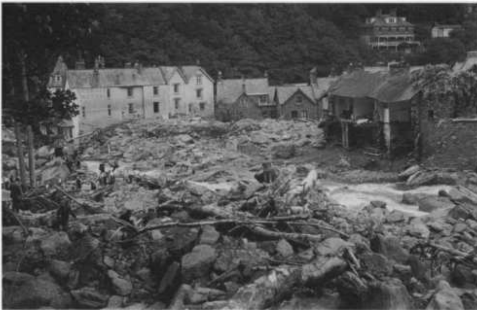
Fig. 1.7 Lynmouth, Devon, after the flood of August 1952. A reminder never to underestimate the power of water. Note the boulders piled against the Lyndale Hotel to a depth of around 9 m, and the water staining on the walls. Midway between the camera and the hotel are many human figures and a bulldozer, which gives some sense of scale. (Reproduced by permission of the Western Morning News , Plymouth)
