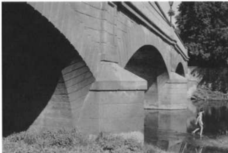
Fig. 1.4 Thomas Telford’s 1831 bridge over the River Wansbeck at Morpeth, Northumberland. Note the cornes de vache at the arch springings.
