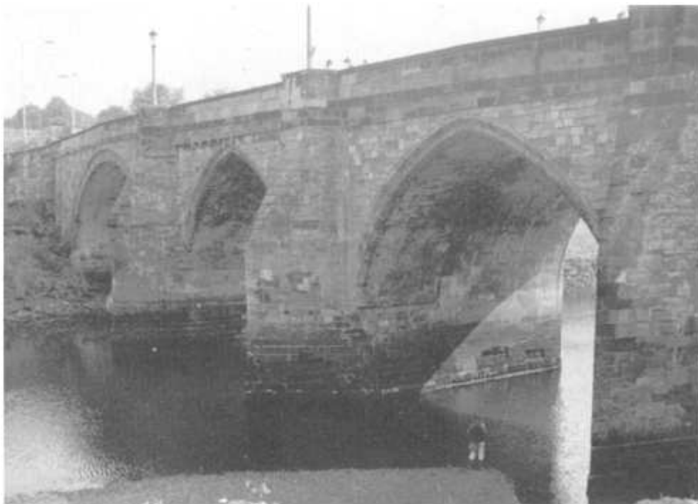
Fig. 1.3 The original fifteenth century part of this bridge across the tidal River Tees at Yarm has characteristic pointed arches (nearest the camera). It was constructed with a road width of about 3.7 m, but this was increased in 1806, the 'join' just being visible. The combination of a spate in the river with a high tide has frequently resulted in the town being flooded to a depth of several metres, notably in 1771 and 1881.
