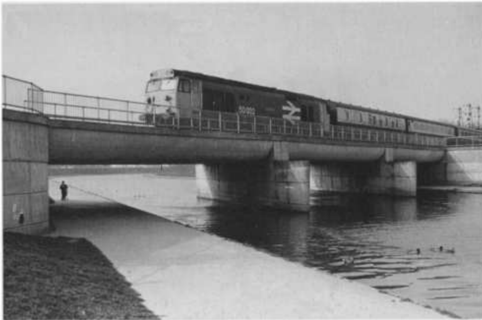
Fig. 1.1 Exwick rail bridge; part of the flood relief channel at Exeter, Devon. Note the rounded soffit and abutments, and elongated piers. A physical hydraulic model study of the scheme was undertaken, and this is to be recommended whenever novel designs or complex flows are involved.
