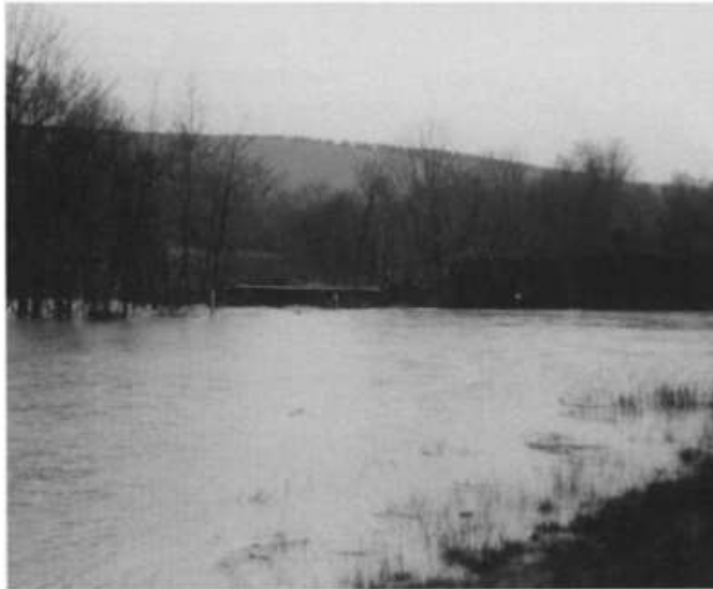
Fig. 2.1 Upstream of Canns Mill Bridge during a 1 in 5 year flood (see also Fig. 2.15 ). The bridge is in the centre of the photo. The width of the floodwater is about 55 m while the bridge span is 4.3 m. The bridge appears to be responsible for the flooding, but only exacerbates it. The primary cause is the low conveyance of the downstream channel. Much of the water on the upstream floodplain is static overbank storage, a fact that must be recognised in any hydraulic analysis. (Photo courtesy of G.A.McInally)
