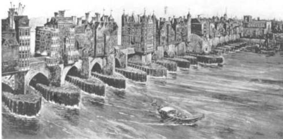
Fig. 1.2 London Bridge was built between 1176 and 1209. The openings are only about half the width of the river, and vary in shape and size. Houses and shops line the bridge. (Copyright © The Musuem of London)
