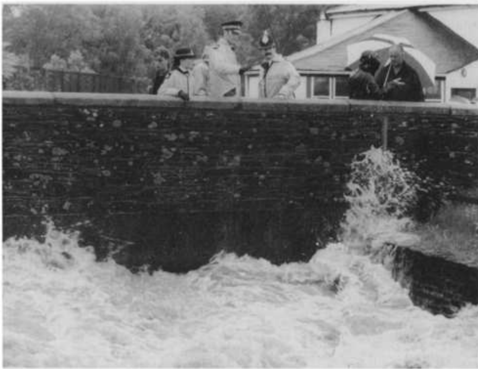
Fig 2.7 There was some concern regarding the safety of this bridge at Camelford in June 1993. Note the extreme turbulence as the opening starts to drown. This illustrates the difficulty of measuring upstream water levels accurately and in determining the height required for an opening to ensure a minimum freeboard of 0.6 m. (Reproduced by permission of Newquay Press Service)
