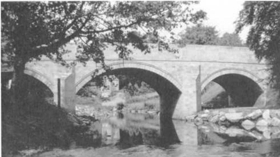
Fig. 1.5 This new three-span masonry bridge across the River Esk at Egton Bridge, North Yorkshire, was opened in 1994, replacing an unattractive 1930s steel structure. The bridge is an exact replica of the original 1758 structure, two spans of which were destroyed by flood in 1930.
