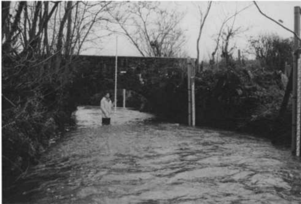
Fig. 2.15 Canns Mill after the flood, showing the water level gauges and flood height (the white mark on the bridge parapet).
