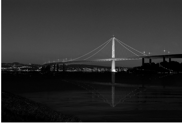
FIGURE 1.18 New eastern spans of the San Francisco-Oakland Bay Bridge.
