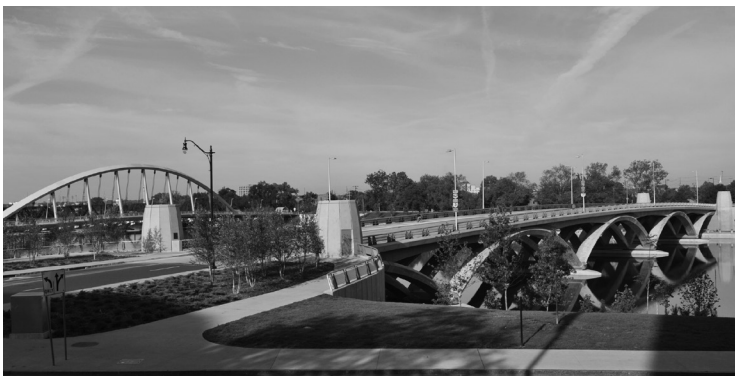
FIGURE 3.17 Two existing traditional bridges, both eligible for the National Register of Historic Places, were replaced by bridges of innovative contemporary design in tune with the community's aspirations and self-image. Rich Street and Main Street Bridges, Civic Center, Columbus, Ohio.
