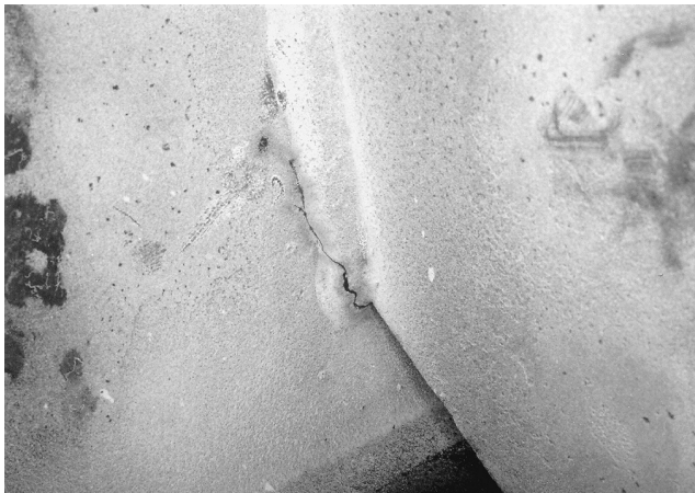
FIGURE 19.7 View of crack in the fillet weld joining the diaphragm connection plate to the web of a box section in the Washington Metro elevated structures. The crack is caused by distortion in the small gap between the bottom of the attachment plate and the box girder flange.
