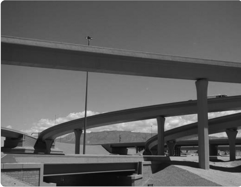
FIGURE 3.14 Albuquerque’s Big I interchange has a theme covering pier shapes, MSE walls, standard details, and colors, the latter developed with community input. (From AASHTO, Bridge Aesthetics Sourcebook , American Association of State Highway and Transportation Officials, Washington, DC, 2010. With permission.)
