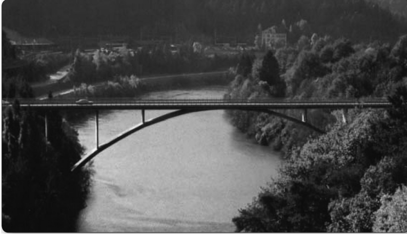
FIGURE 3.6 Rock foundations permit arch bridges. Christian Menn's Reichenau Bridge, Switzerland. (From AASHTO, Bridge Aesthetics Sourcebook , American Association of State Highway and Transportation Officials, Washington, DC, 2010. With permission.)
