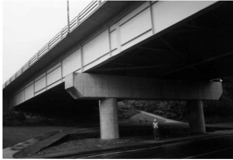
FIGURE 16.14 Rehabilitated columns of the Portage Creek Bridge in British Columbia, Canada.
