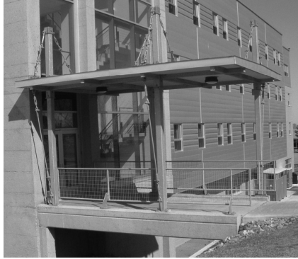
FIGURE 16.24 Université de Sherbrooke Pedestrian Bridge. (From ISIS, Design Manual 3: Reinforcing Concrete Structures with Fibre Reinforced Polymers . ISIS Canada, Intelligent Sensing for Innovative Structures, A Canadian Network of Centres of Excellence, University of Manitoba, Winnipeg, Manitoba, Canada, 2007a. With permission.)
