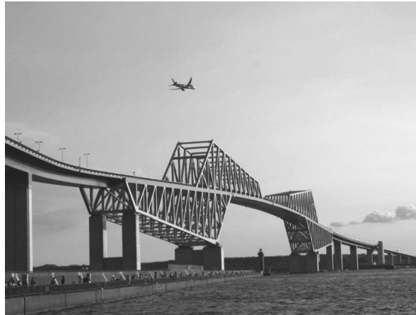
FIGURE 17.2 Tokyo Gate Bridge.
