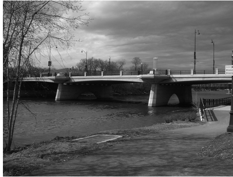
FIGURE 3.23 Rather than pasting bulky, vaguely historical ornament on a conventional structure, the designers of the Wilson Street Bridge in Batavia, Illinois have dealt with a historic setting in a different way. They have combined a structure of amazing thinness, only possible because of modern high strength concrete and post tensioning, with traditional details that reflect the nature of its setting. Both the past and the future are expressed, whereas views up and down the river are reopened that had been blocked for decades by the previous earth-filled concrete arch.
