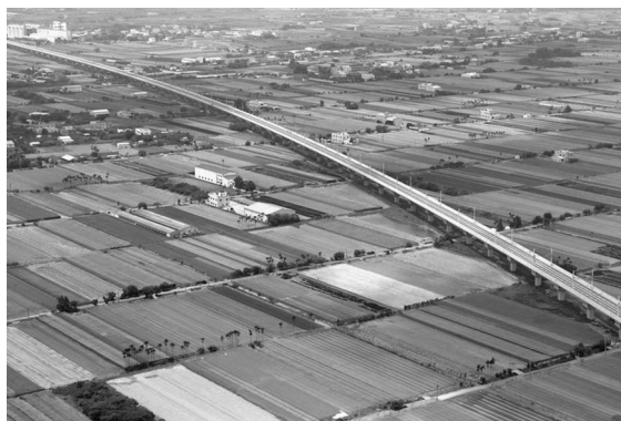
FIGURE 8.1 Aerial photo of Taiwan high-speed rail elevated viaduct.
