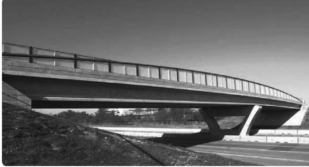
FIGURE 3.22 This pedestrian fence uses standard chain link, but the arched top edge, carefully designed details and distinctive color improve the appearance of the bridge without a significant increase in cost, I-235 Reconstruction, Des Moines, Iowa ( Sourcebook 4–24). (From AASHTO, Bridge Aesthetics Sourcebook , American Association of State Highway and Transportation Officials, Washington, DC, 2010. With permission.)
