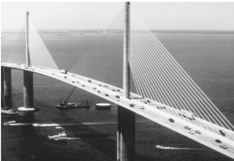
FIGURE 3.8 The Sunshine Skyway.
