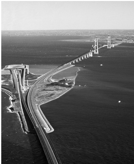
FIGURE 4.5 The Great Belt Fixed Link. Combined road and rail low-level West Bridge in foreground, East Bridge suspension road bridge, and ramp to the East Tunnel for railway. (Courtesy of Sund & Bælt Holding A/S.)
