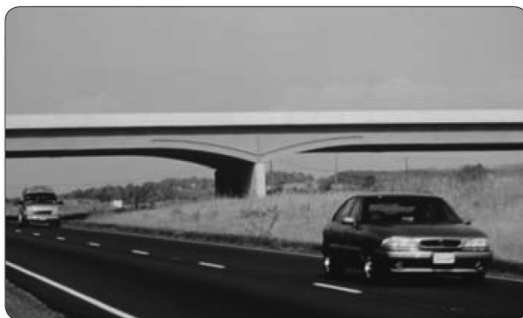
FIGURE 3.18 The haunch gives this girder a more interesting and attractive shape that also tells a story about the flow of moments and forces in the structure. The stiffener is utilitarian but its placement and curvature make it ornamental as well, so that it reinforces the story told by the haunch. I-81, Virginia. (From AASHTO, Bridge Aesthetics Sourcebook , American Association of State Highway and Transportation Officials, Washington, DC, 2010. With permission.)
