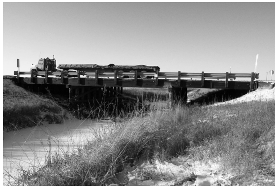
FIGURE 16.25 Tourand Creek Bridge in Manitoba, Canada.
