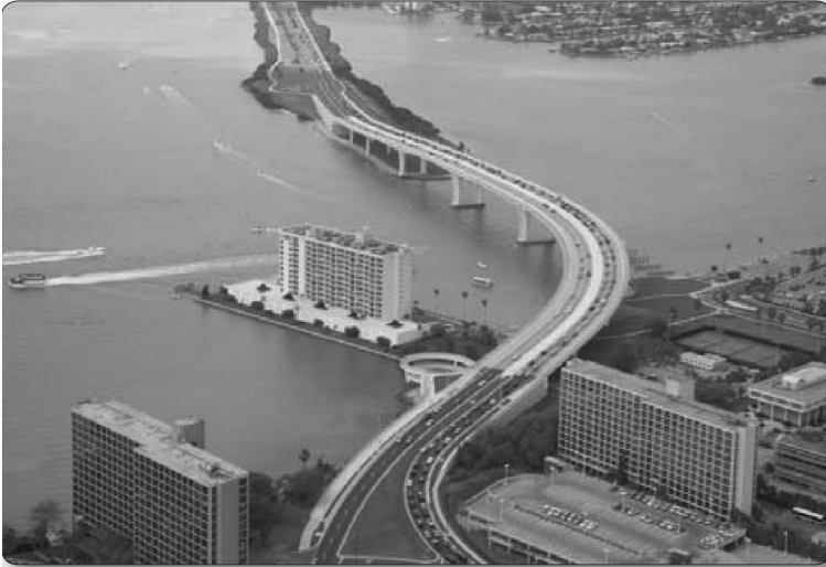
FIGURE 3.16 An example of a successful collaboration between an engineer and an architect/urban designer which considers nearby land uses and views as well as technical requirements. Clearwater Memorial Causeway, Clearwater, Florida. (From AASHTO, Bridge Aesthetics Sourcebook , American Association of State Highway and Transportation Officials, Washington, DC, 2010. With permission.)
