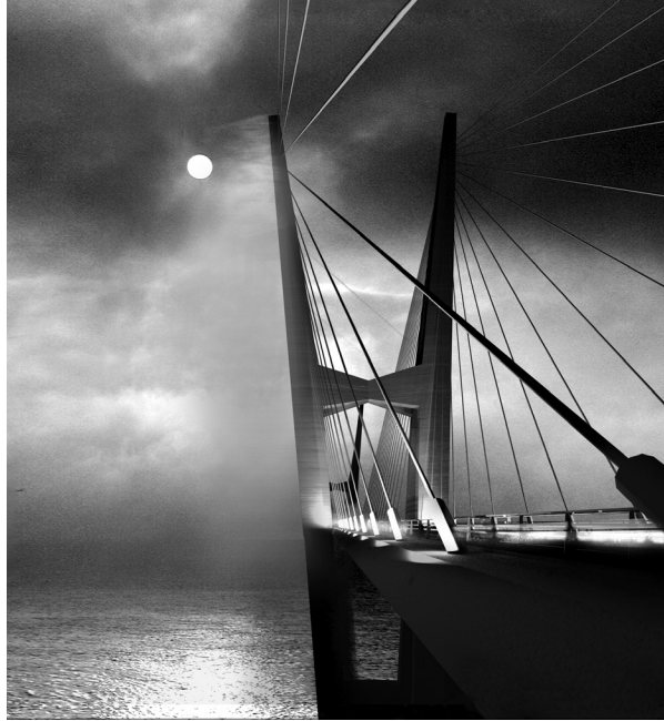
FIGURE 4.2 Fehmarnbelt conceptual design for cable-stayed bridge for road and rail. Example of project with landmark quality. (Courtesy of Dissing+Weitling architecture.)
