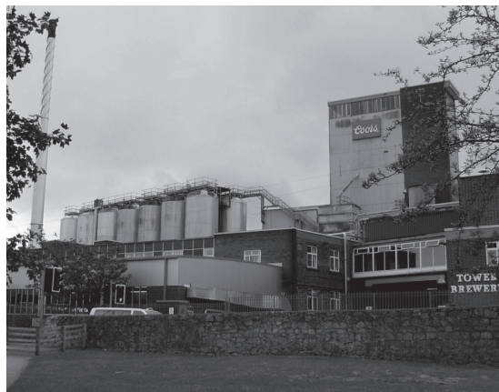
(d) Large cylindrical brewing/maturation vessels at Coors Brewery, Tadcaster, UK.
