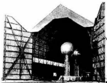
*Figure 23 – Ten million volt Van de Graaff generators were built in the 1930's. One generator here is negatively charged, and the other is positive. Generators of this size are not recommended as a first project. (Perhaps not even as a second! ...but call me if you build one!)*
