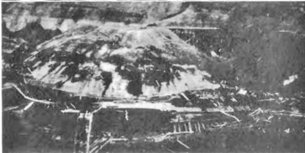
The gigantic V-2 storage bunker at Wizernes, France after absorbing 14 Allied air attacks. Today the bunker is a museum run by the French government called La Coupole. It contains originals of the V-1 and V-2 and also celebrates space travel. Carefully considered German camouflage schemes were designed to conceal the weapons among trees.
