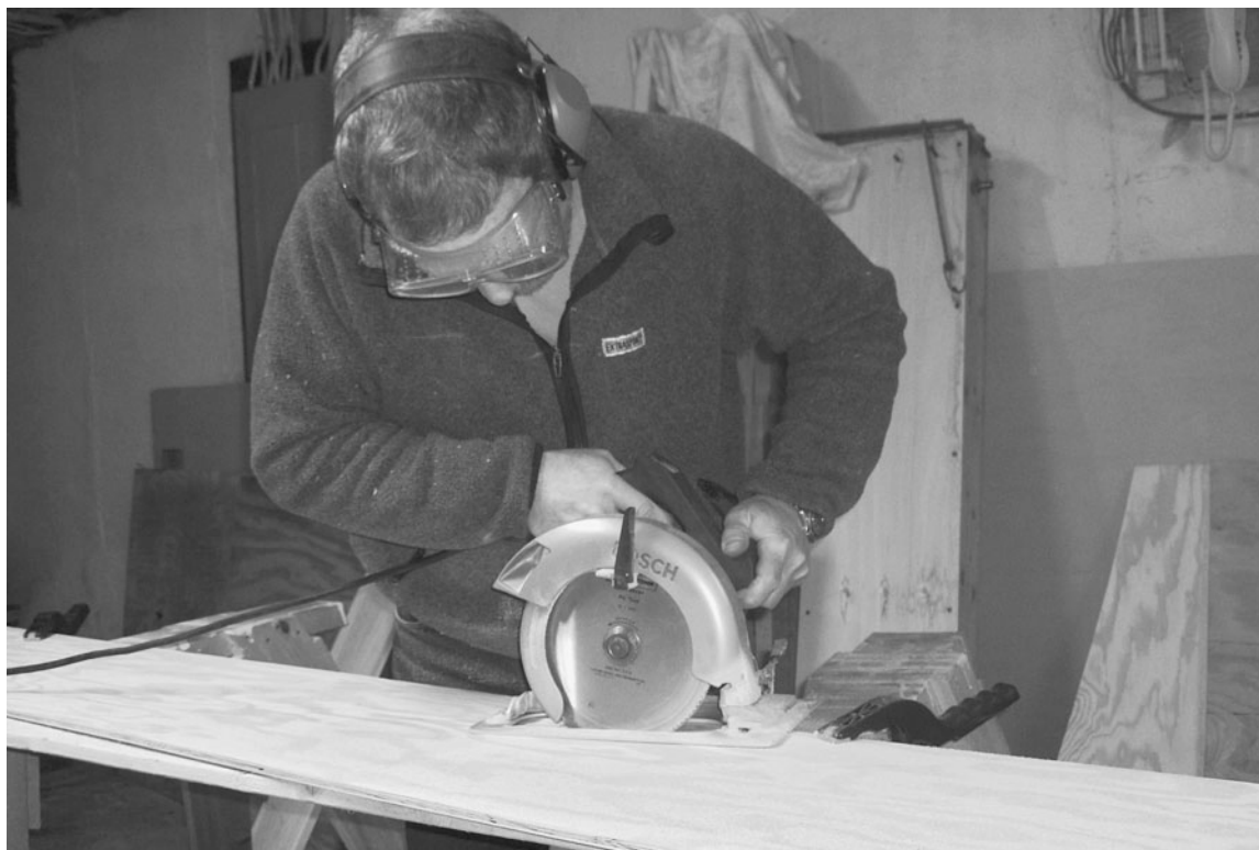
Cutting out the long plywood panels with a circular saw. It's possible to cut fair curves with a circular saw by setting the blade just deep enough to break through the bottom of the plywood. Note the long pieces of lumber below the plywood, which are used to support it in the middle of the span between the sawhorses. (Maxwell Holtzman)
