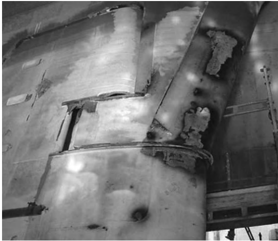
FIGURE 11.7 Example of rudder erosion.
