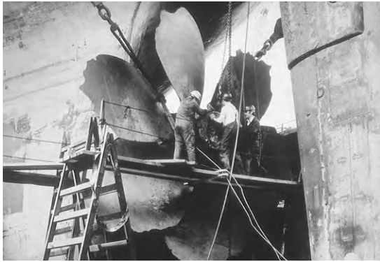
FIGURE 26.3 Propeller damage due to impact damage with mooring chains.
