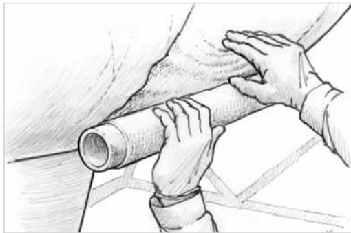
Figure 3. Unroll the fiberglass onto the surface with one hand—spread out wrinkles and press the fabric against the surface with the other.
