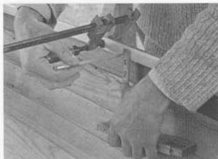
Marking the frame centerlines on the sheer clamp.
