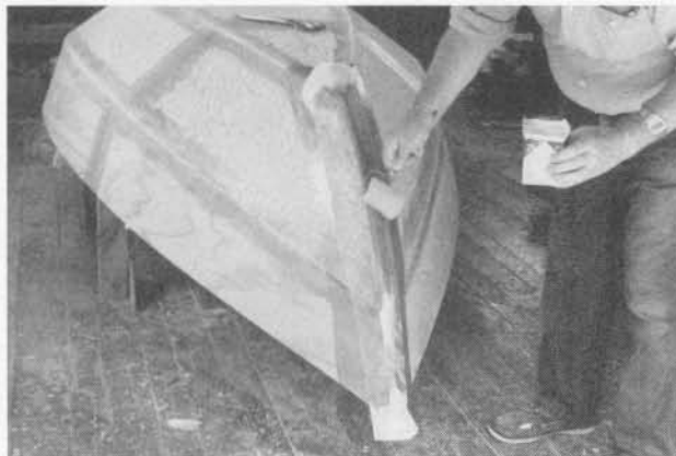
Lay the stem tape or cloth into wet resin and wet it out with more resin until it lies smoothly in all directions and the weave is filled.
