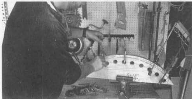
Simple jigs are used to laminate the deckbeams.
