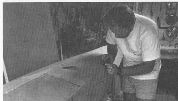
After turning the hull over, cut off the tie-wires, sand off any epoxy that's dripped through the edges, and clean up the outside seams with a plane.
