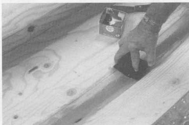
Try to make a smooth fillet along the long inside seams.
