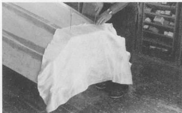
Cut a piece of 10-ounce cloth for a generous fit over the transom.
