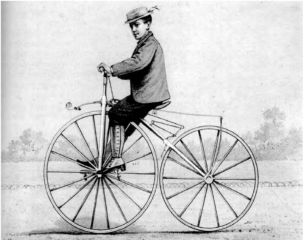
Figure 8.3 A machine with a block and tackle below the saddle, which increased the amount of force that could be applied to the brake ( Le Centaure , September 1868).
