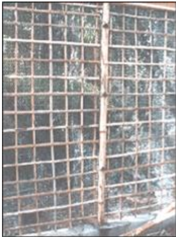
< Figure 17- Grids of split bamboo constructed between bamboo poles (Image courtesy of IPIRTI - Bangalore, India)
