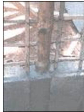
< Figure 17- Grids of split bamboo constructed between bamboo poles (Image courtesy of IPIRTI - Bangalore, India)
