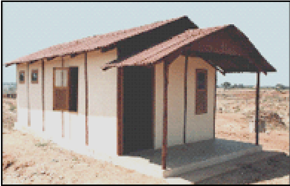
Figure 12- Prototype of a Bamboo house constructed according to the above technology (Image courtesy of IPIRTI - Bangalore, India)
