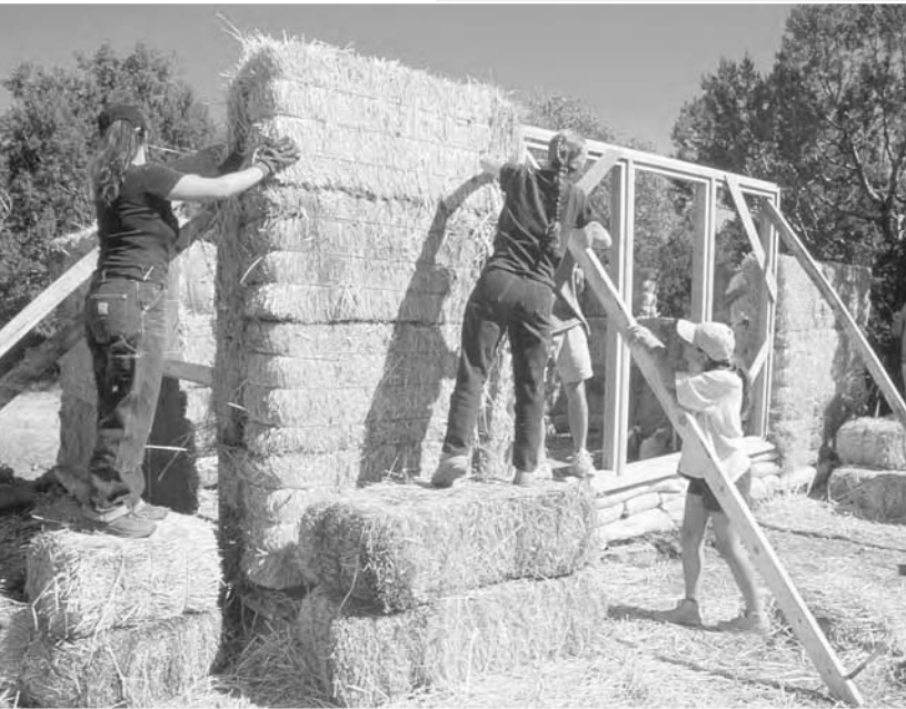
3-8: An affordable straw bale house prototype, under construction in New Mexico. This house features a low-tech, recycled concrete and earthbag foundation, straw bale walls with earth plasters, and a simple metal roof supported by pallet trusses.
