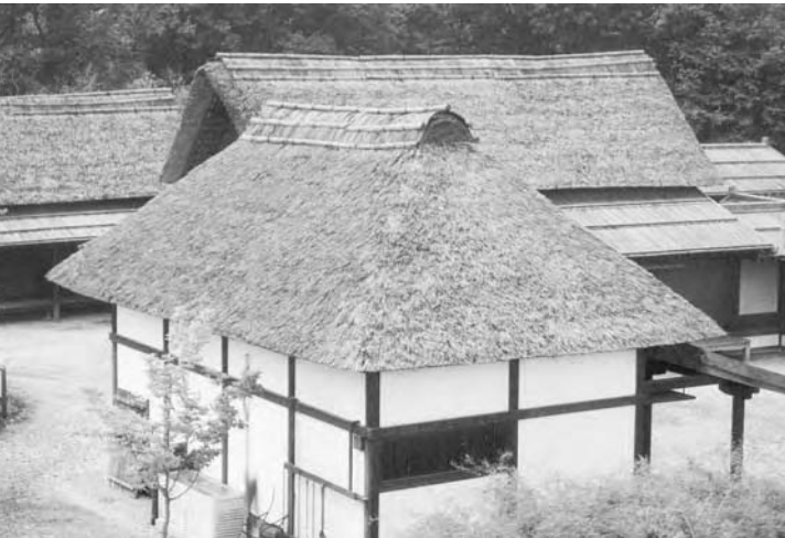
7-5: A traditional village in Japan demonstrates timber framing, wattle and daub infill, limewash, and thatched roofs.
