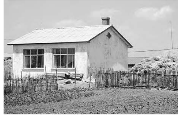
4-6: A completed brick and straw bale house. Note its passive solar orientation, lime-plastered walls, and conventional roof.
