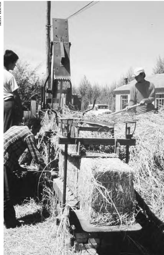
3-4: Simple machinery, such as this baler in China, can be used to create building materials from local resources. The resulting straw bales are inexpensive, relatively easy to build with, and highly insulating.
