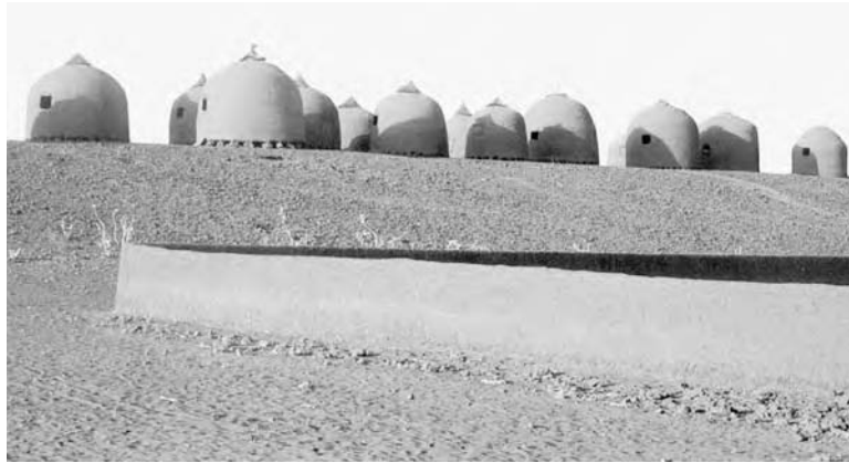
2-3: Granaries in Affala, Niger are built in coils, an application of a pottery-making technique on a larger scale.
