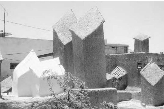
3-3: Wind catchers in Tatta, Pakistan. Reaching up from the roof, wind catchers capture cooling breezes and channel them down into the house.
