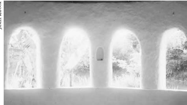
2-9: The use of cob, a sculptural earthbuilding technique that results in monolithic walls, allows for such beautiful details as these arched windows for this bahn din (mud house) at Wongsanit.
