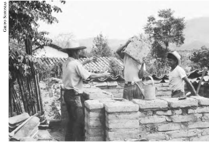
6-6: Community members building a house, using adobe bricks.
