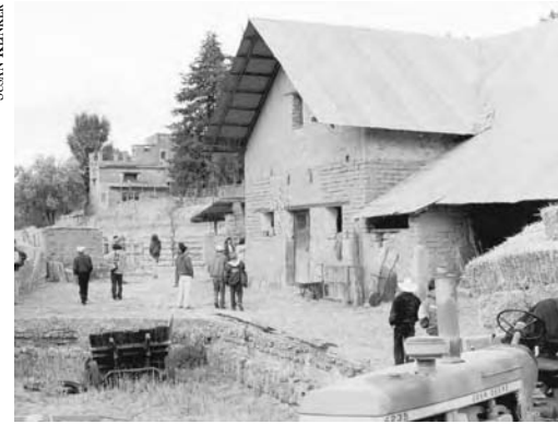
4-8: By visiting traditional earthen buildings in the region near Zopilote, students gain a sense of history, as well as the technological information necessary for developing innovations.
