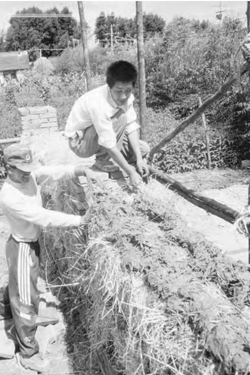
4-2: Mud is used to stabilize relatively soft bales.
