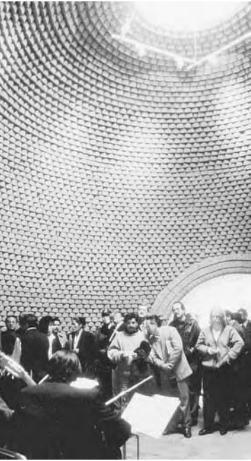
7-19: The interior of an adobe house in La Paz, Bolivia. Note the articulation of adobes on the inner surface for better acoustic performance.
