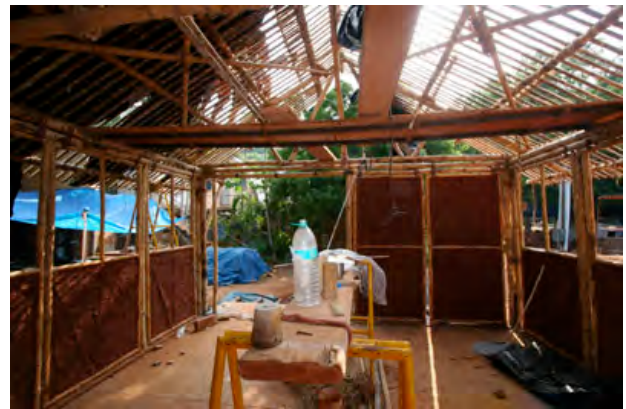
Figure 17 - Panels with one layer of daub placed in the structure
