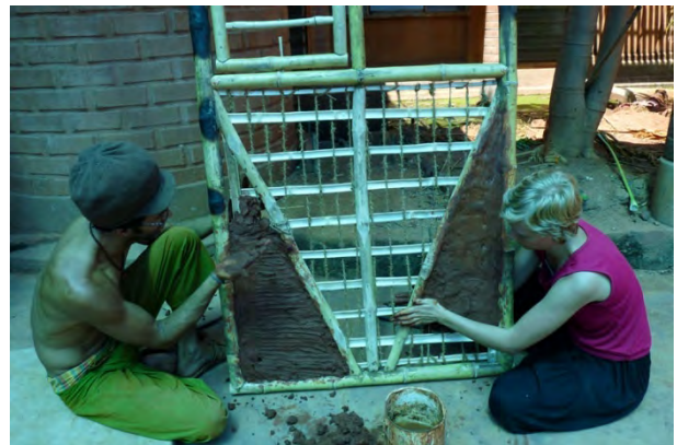
Figure 9 - Applying the first layer of daub
