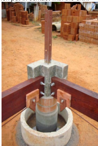
Figure 10 - Floor beams and tension rods added
