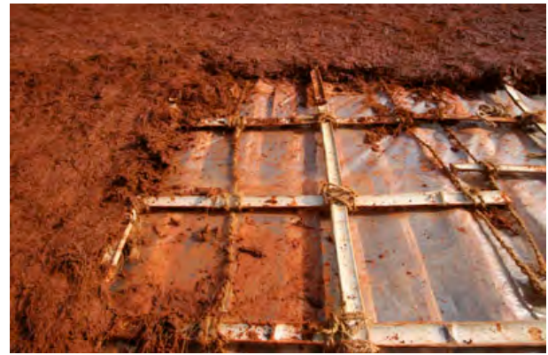
Figure 21 - Mud plaster layer (5cm thick)
