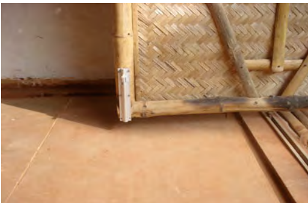
Figure 29 – View of the door
