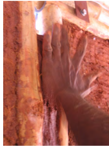
Figure 19 - Filling the gaps
