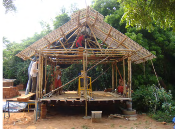
Figure 16 - Roof substructure nearly complete
