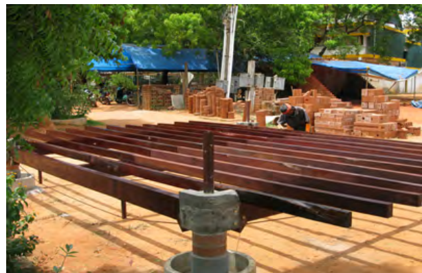
Figure 11 - Floor substructure
