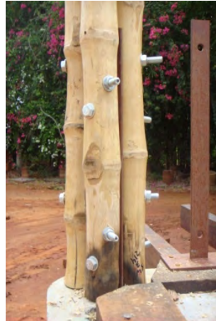
Figure 12 - Posts fixed with bolts
