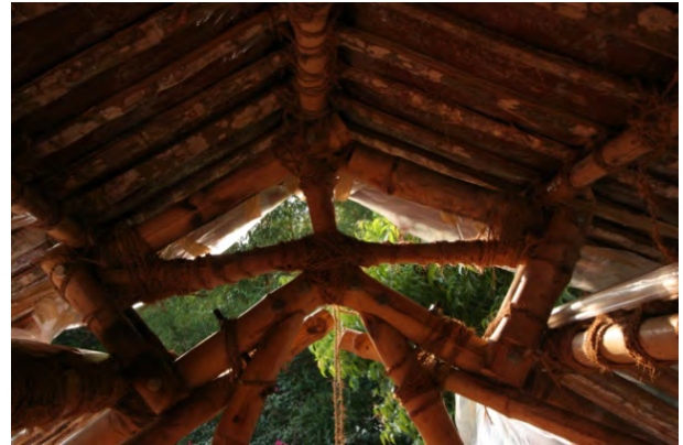
Figure 7 - Truss ridge crown modification
