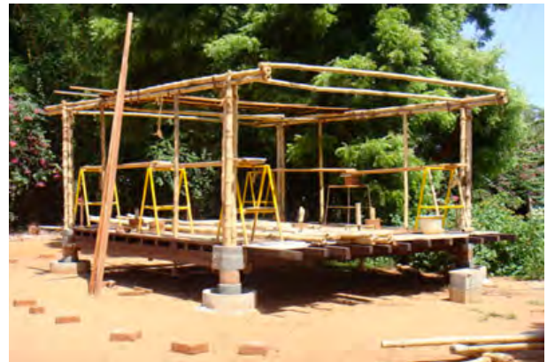
Figure 14 - Posts and beams
