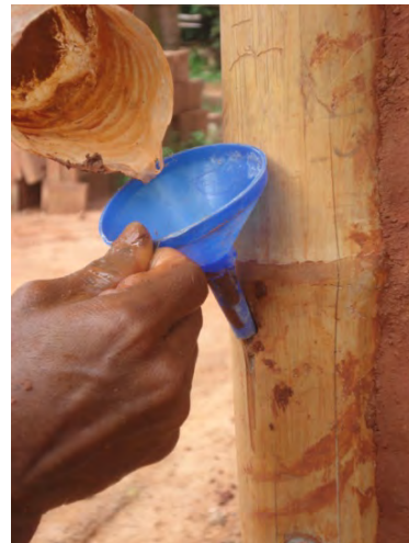
Figure 18 - Cement poured into post. A larger funnel than pictured is recommended
