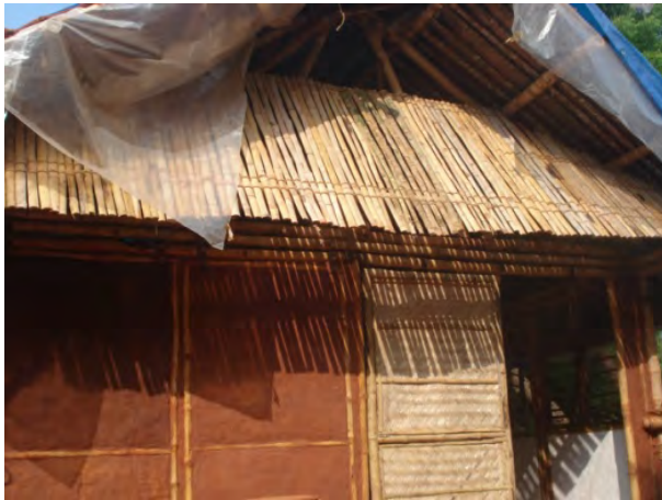
Figure 26 - Eave exterior view
