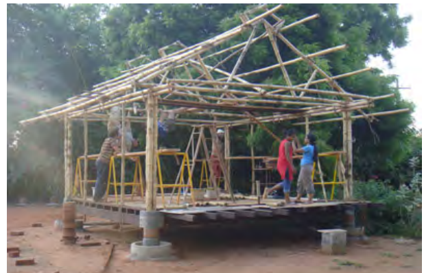
Figure 15 - The purlins in place
