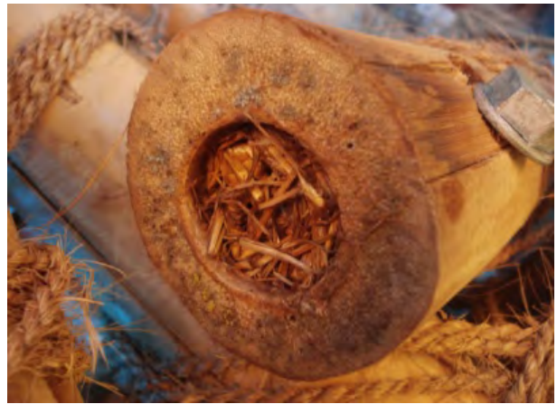
Figure 23 - Ends filled to prevent rodent habitation
