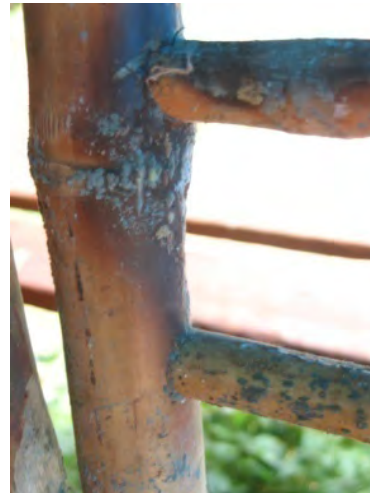
Figure 32 - Mould during the monsoon
