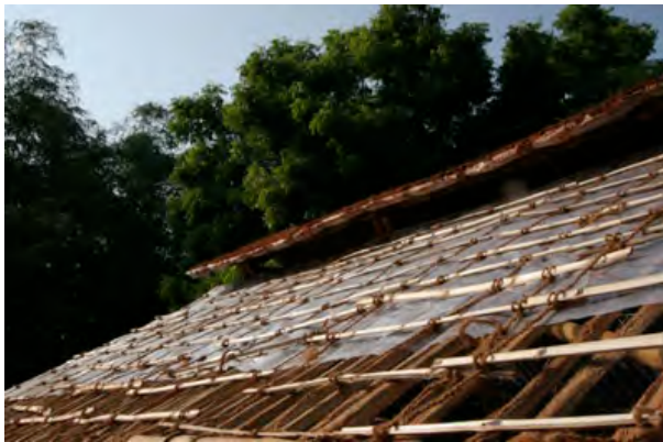
Figure 20 - Plastic sheet and lattice of bamboo and coconut rope
