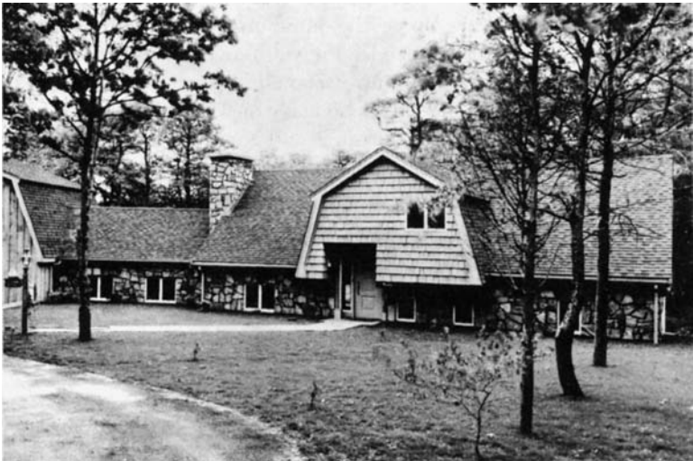
Figure 15-10 Wood shingles blend well with stone veneer on this home.
