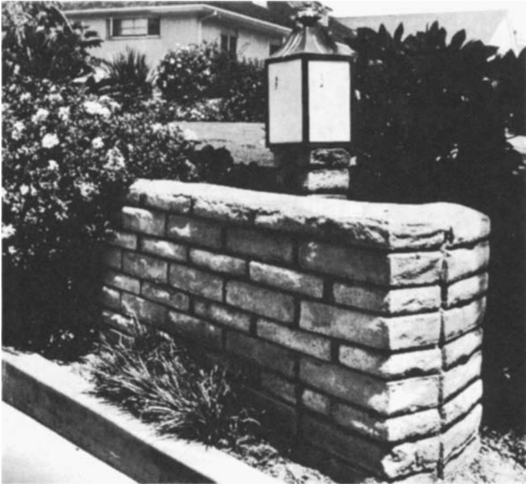
Figure 5-5 A wall of slump block adds rustic charm and is especially suitable for ranch-type homes.
