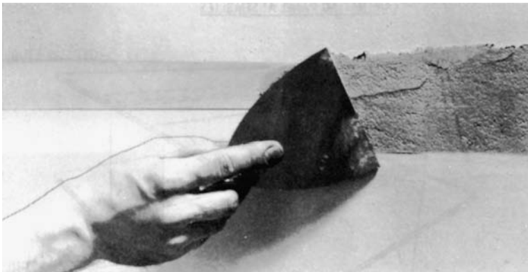
Figure 18-25 The first step in finishing joints between plasterboard. (Courtesy National Gypsum Co.)
