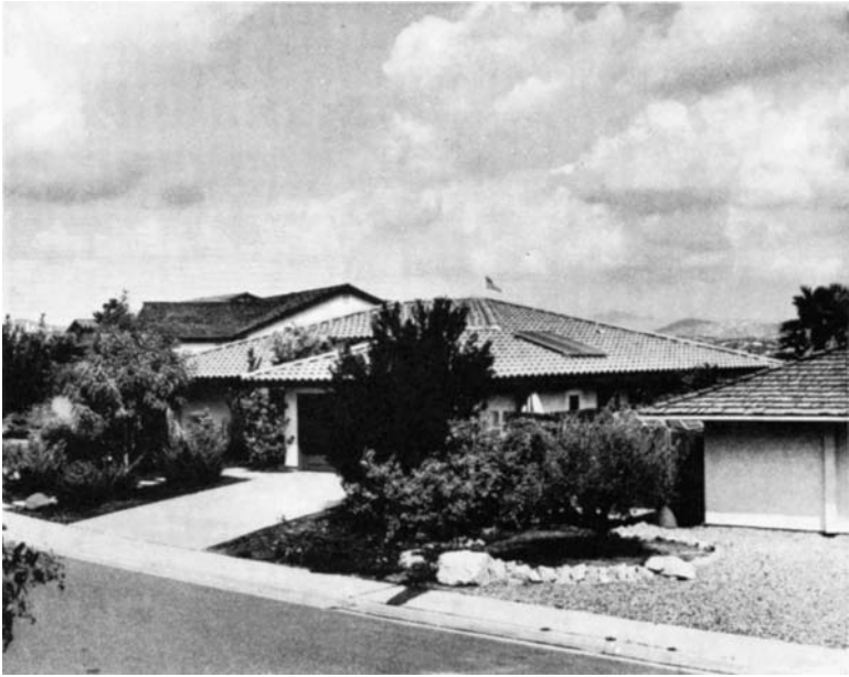
Figure 13-2 A tile roof. This roof is popular in southwestern states.
