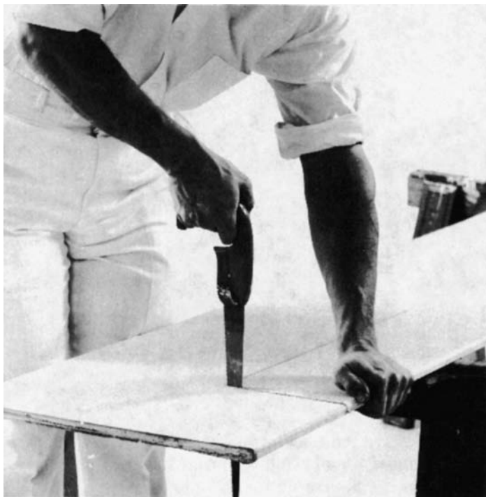
Figure 18-37 Cutting vinyl-covered wallboard for other openings.
