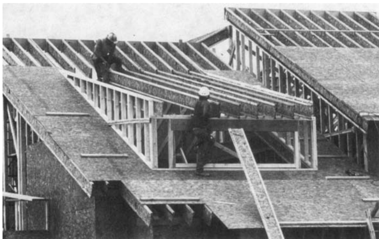
Figure 10-9 Louisiana-Pacific's I-joint used as rafters, and GluLam used as a header. (Courtesy Louisiana-Pacific)
