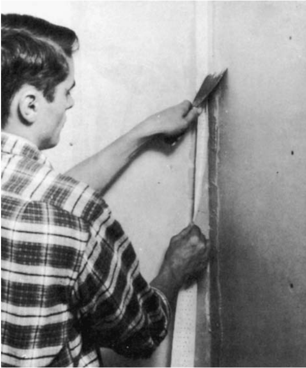
Figure 18-31 Inside corners are handled in the same manner as flat joints. A specially shaped corner knife is also good. (Courtesy National Gypsum Co.)
