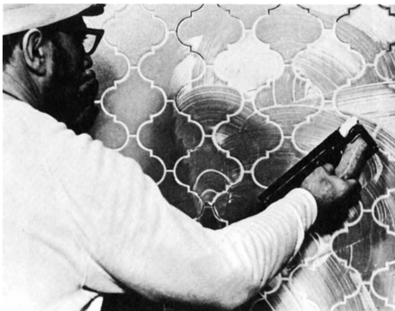
Figure 22-12 A squeegee or rubber trowel is good for smoothing grout.
