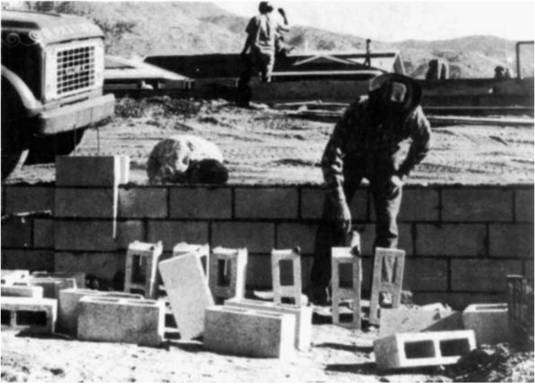
(A) Several blocks are receiving mortar on the end.
