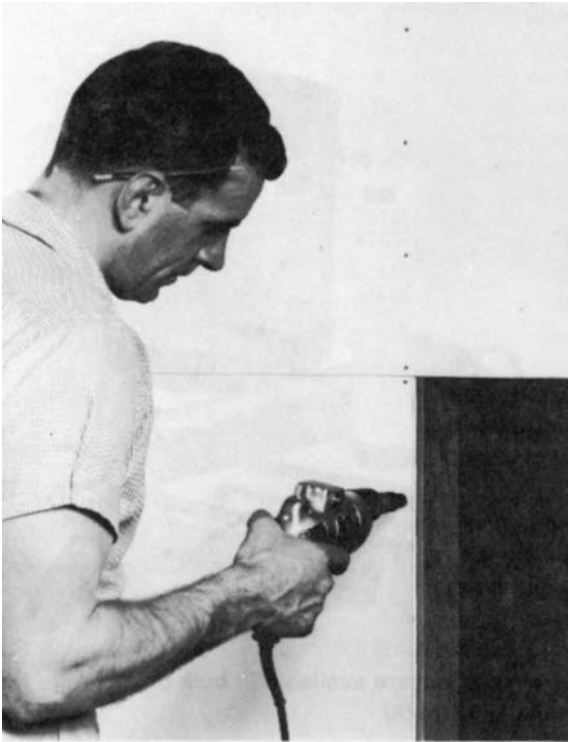
Figure 18-4 Wallboard fastened to studs with a power screwdriver.
