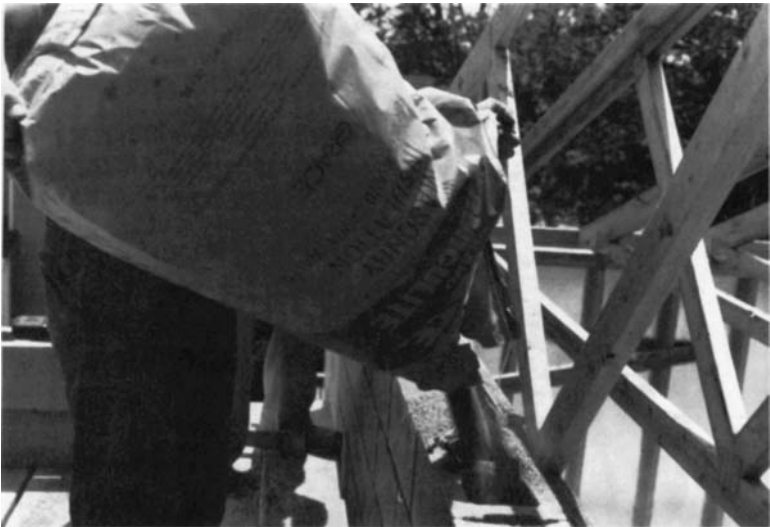
Figure 17-10 Zonolite being installed in concrete blocks.
