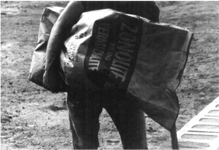
Figure 5-31 Zonolite insulation used to fill cavity in concrete block. (Courtesy W. R. Grace)
