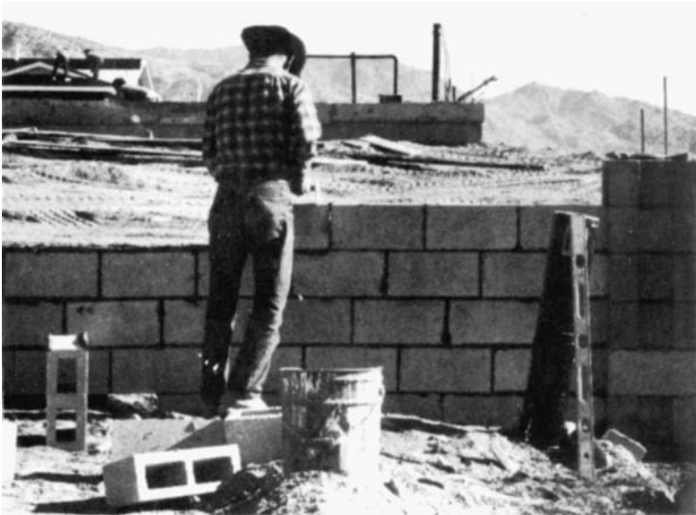
(B) Blocks are tapped into position.
