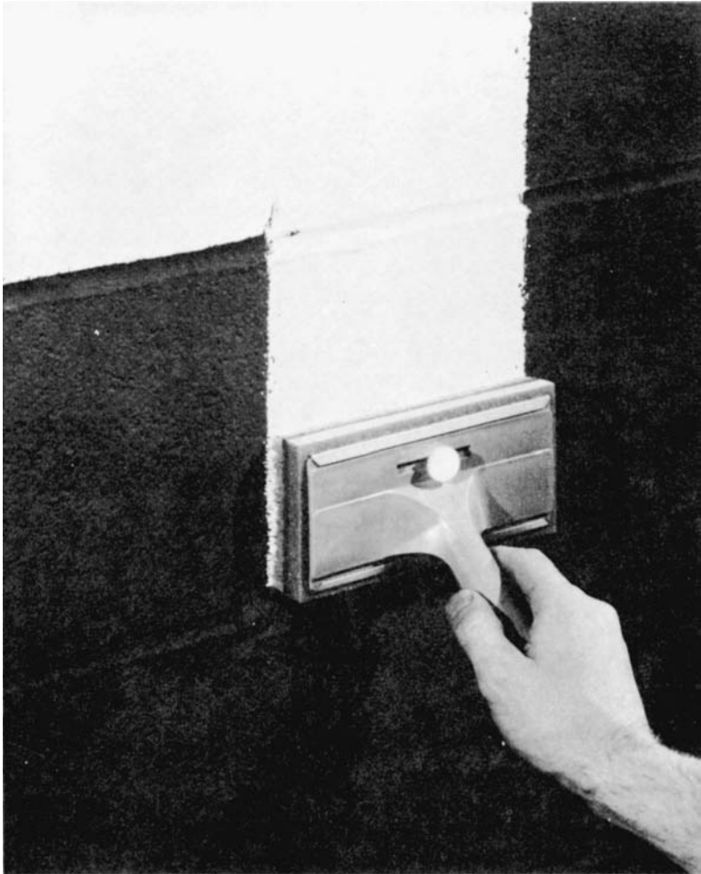
Figure 5-34 Block with V-joints. Block can be painted—pad painter works well on it.
