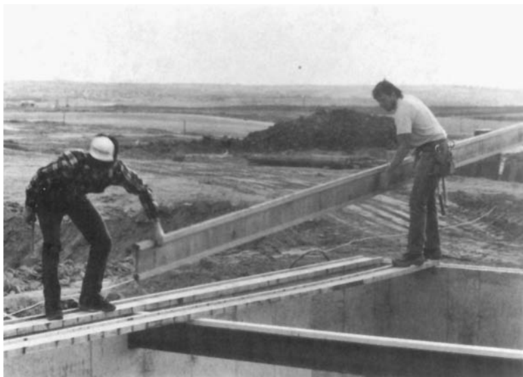
Figure 10-6 TJI joists are available in long lengths to accommodate multiple spans. (Courtesy Trus Joist Corporation)
