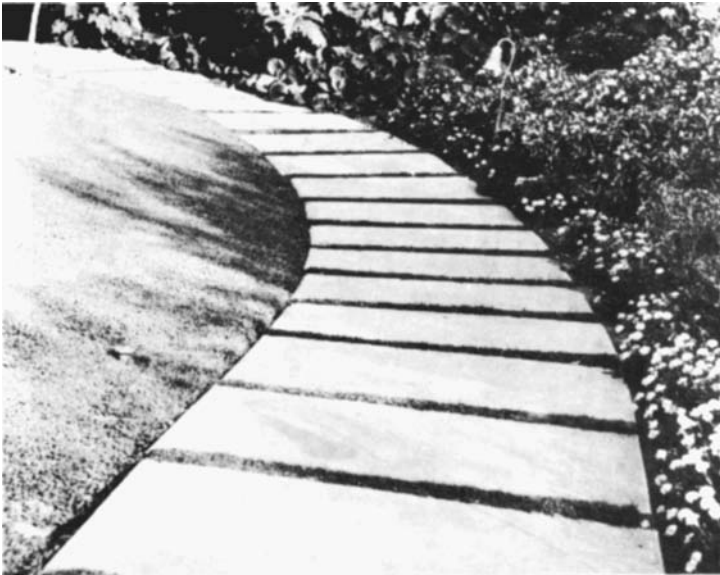
Figure 5-13 Extra-large precast concrete slabs used to make an attractive walk.
