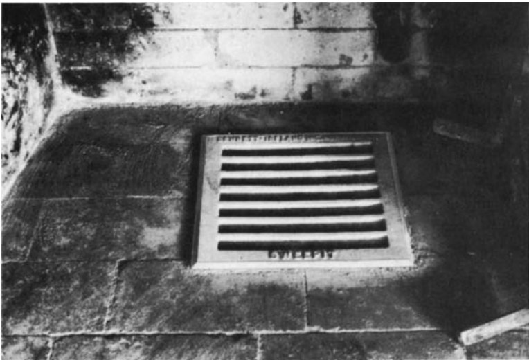
Figure 6-14 A cast-iron grate over the ash box to keep large pieces of burning wood from falling into the ash box.
