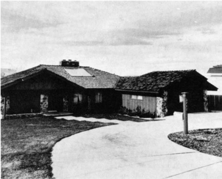
Figure 13-1 A wood shingle roof.
