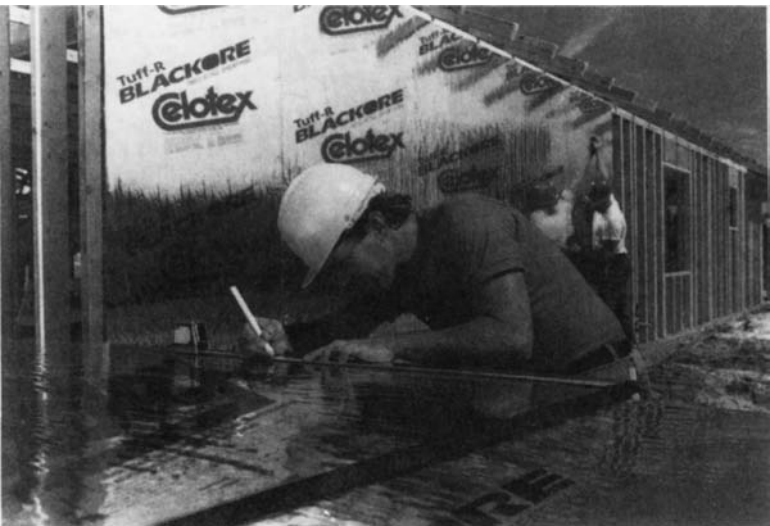
Figure 17-7 Celotex's New Blackore with an R-value of R-8.7 per inch.
