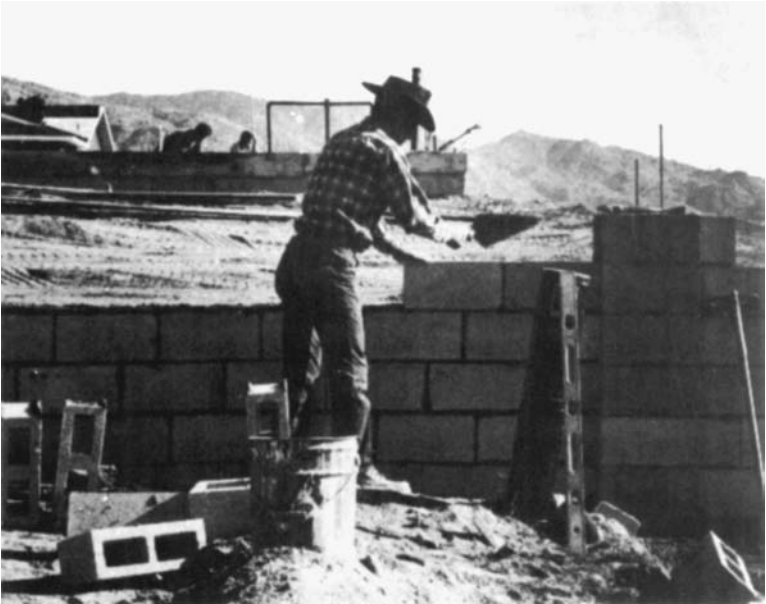
(C) Excess mortar is removed and alignment checked.
