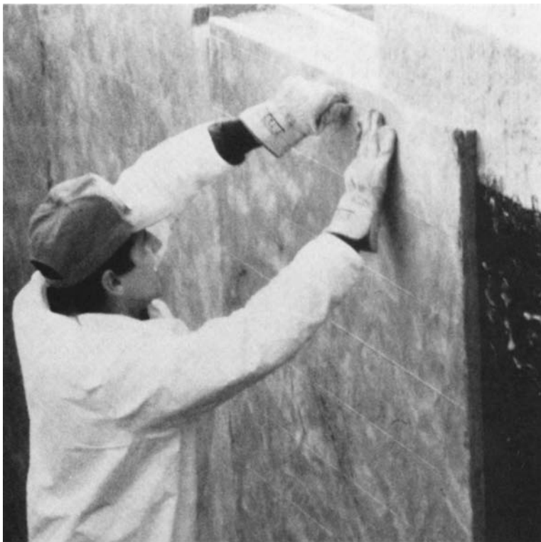
Figure 3-15 Fiberglass drain screen. (Courtesy of Koch Materials Co.)
