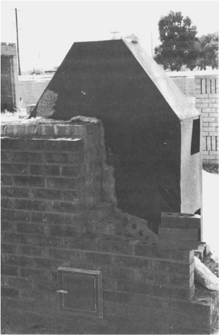
Figure 6-17 Brickwork around the back of a fireplace form.
