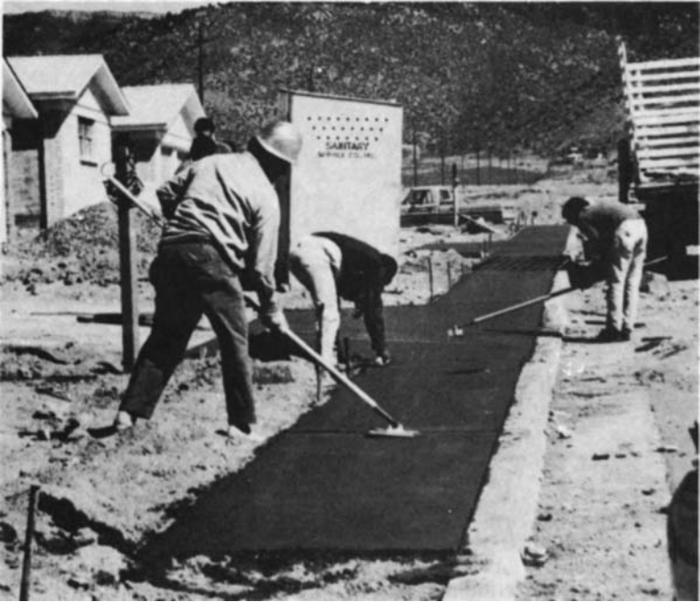
Figure 4-8 Putting the finish on a concrete sidewalk.
