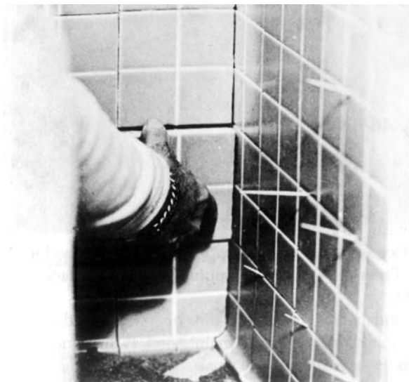
Figure 22-8 If tile does not have spacers, you must provide them.
