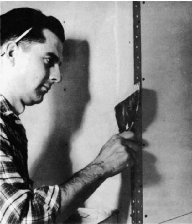
Figure 18-33 Applying compound over the corner bead. (Courtesy National Gypsum Co.)
