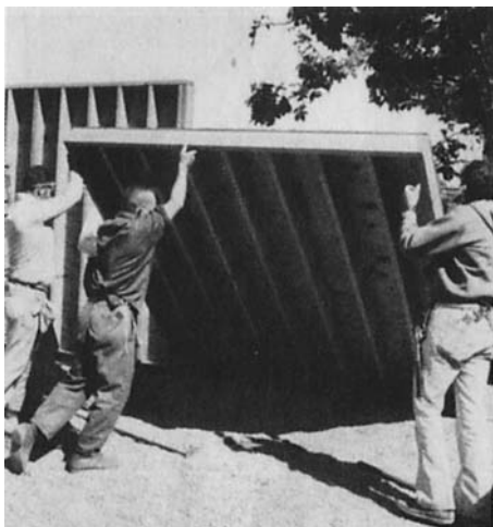
Figure 3-23 Prefab wall sections being erected.
