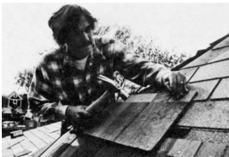
Figure 13-13 Wood fiber roofing from Masonite is a relatively new product. It is available in fire-rated versions and is bigger than standard shingles.
