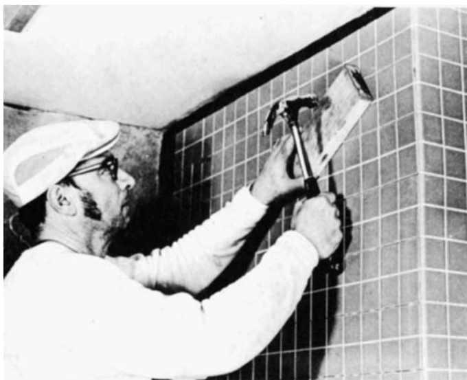
Figure 22-9 Tap tile carefully using a beater block to be sure it is seated properly.
