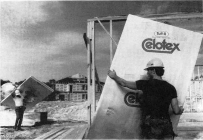
Figure 17-6 Celotex Tuff-R rigid board insulated sheathing.
