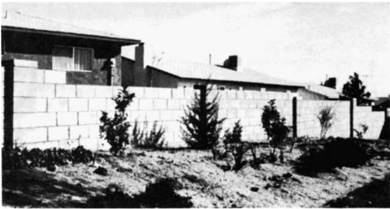
Figure 5-17 A garden wall of concrete blocks. The columns are spaced 15 feet apart.
