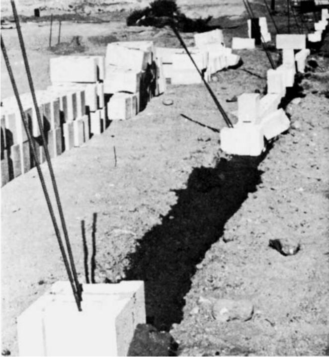
Figure 5-15 Vertical reinforcement rods through double-thick column blocks.
