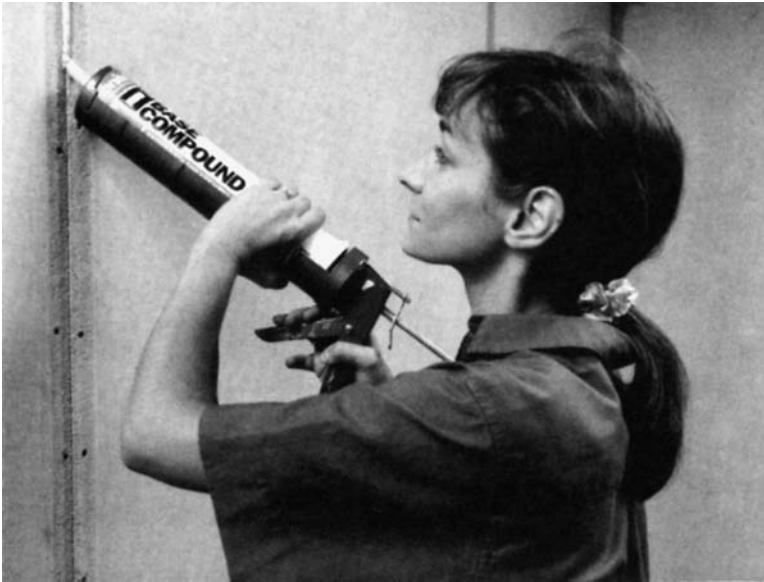
Figure 18-48 Applying caulk glue to Gypsonite panels. (Courtesy Highland American Corporation)
