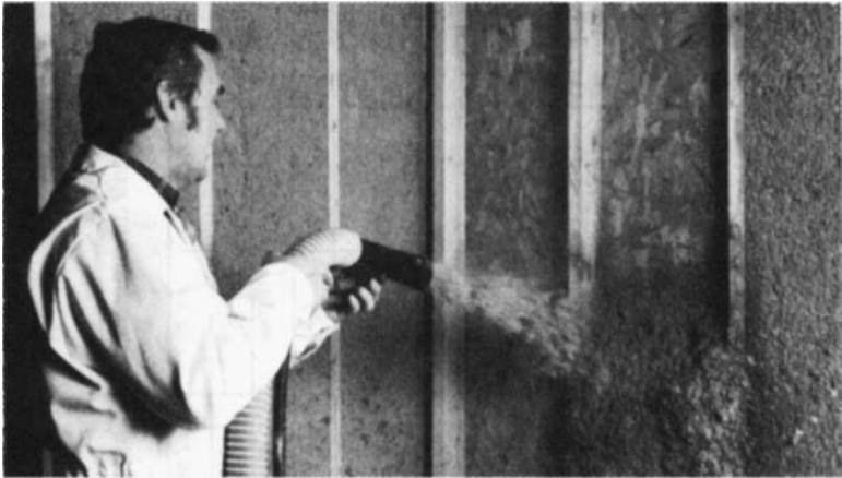
Figure 17-5 Installation of wet-spray cellulose.
