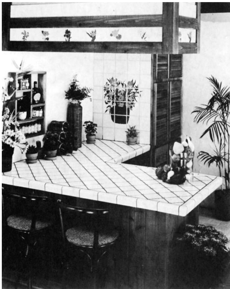
Figure 22-3 Tile is also used for countertops.
