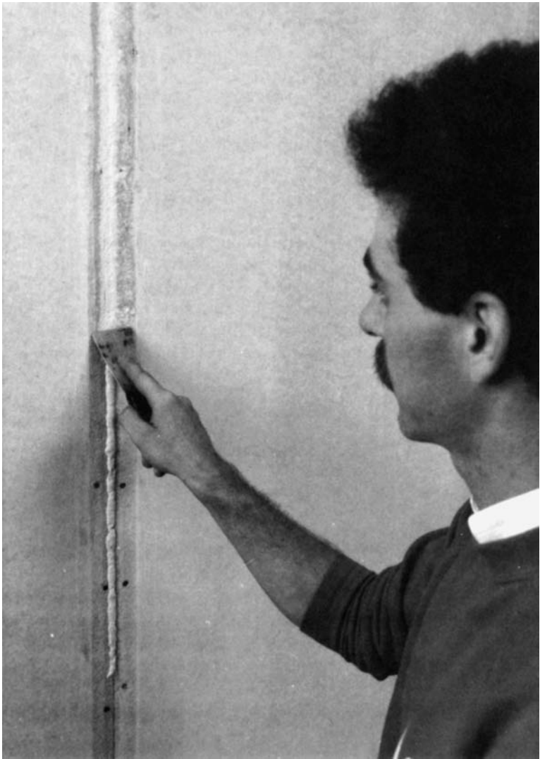
Figure 18-49 Spreading the compound with a putty knife. (Courtesy Highland American Corporation)
