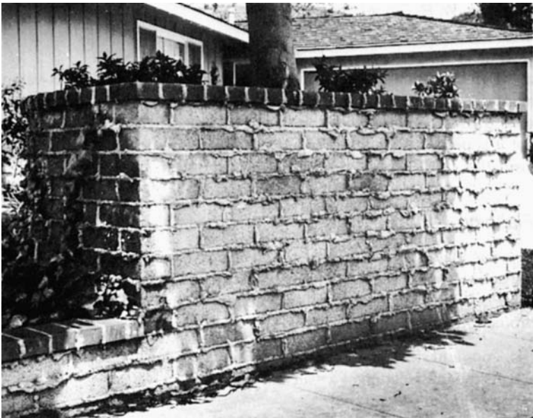
Figure 5-33 Brick wall with extruding joint construction.
