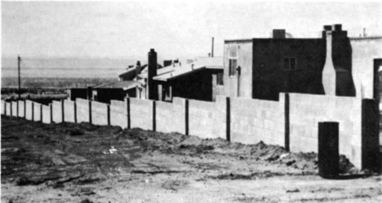
Figure 5-16 A newly finished concrete-block wall. Note reinforcement columns at various intervals.
