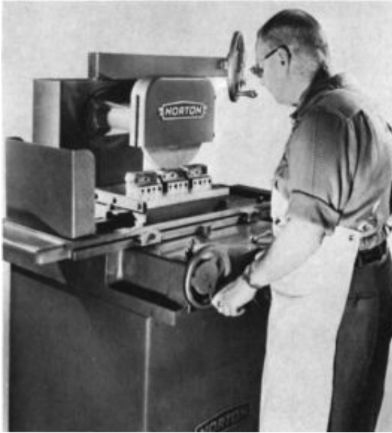
Figure 7-26 Hand-operated surface grinder. (Courtesy Norton Co.)
