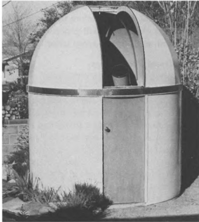
An attractive 8-foot observatory built of plywood and \frac{1}{8} -inch tempered Masonite. It contains a sturdily mounted 8-inch f/6 equatorial Newtonian telescope. (Observatory and photo by Charles Wierzbichi)
