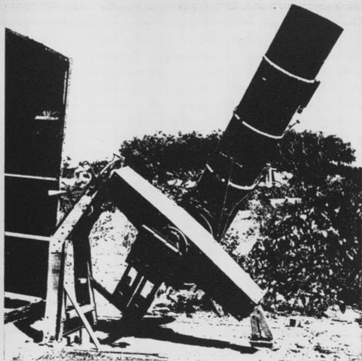
Fig. 112. 330mm (13-inch) equatorial built by G. Gauthier.
