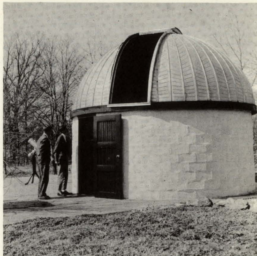
This 17-foot observatory was built by a group of 14- to 17-year-old boys with no outside help. The base is cinder block, surmounted by a converted silo top with hemispheric slide. It holds a 12-inch telescope.
