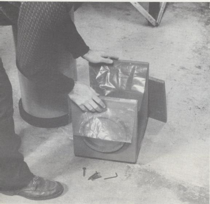
Installing the Tube Step 1: Drape plastic over the tube box.
