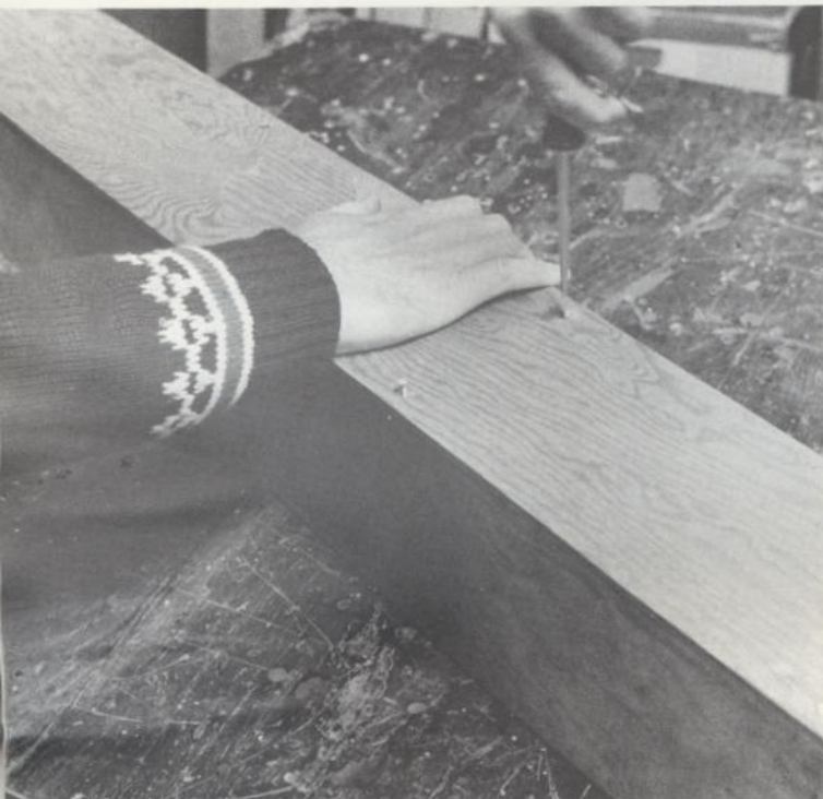
Remove the fourth side in preparation for sealing and painting.
