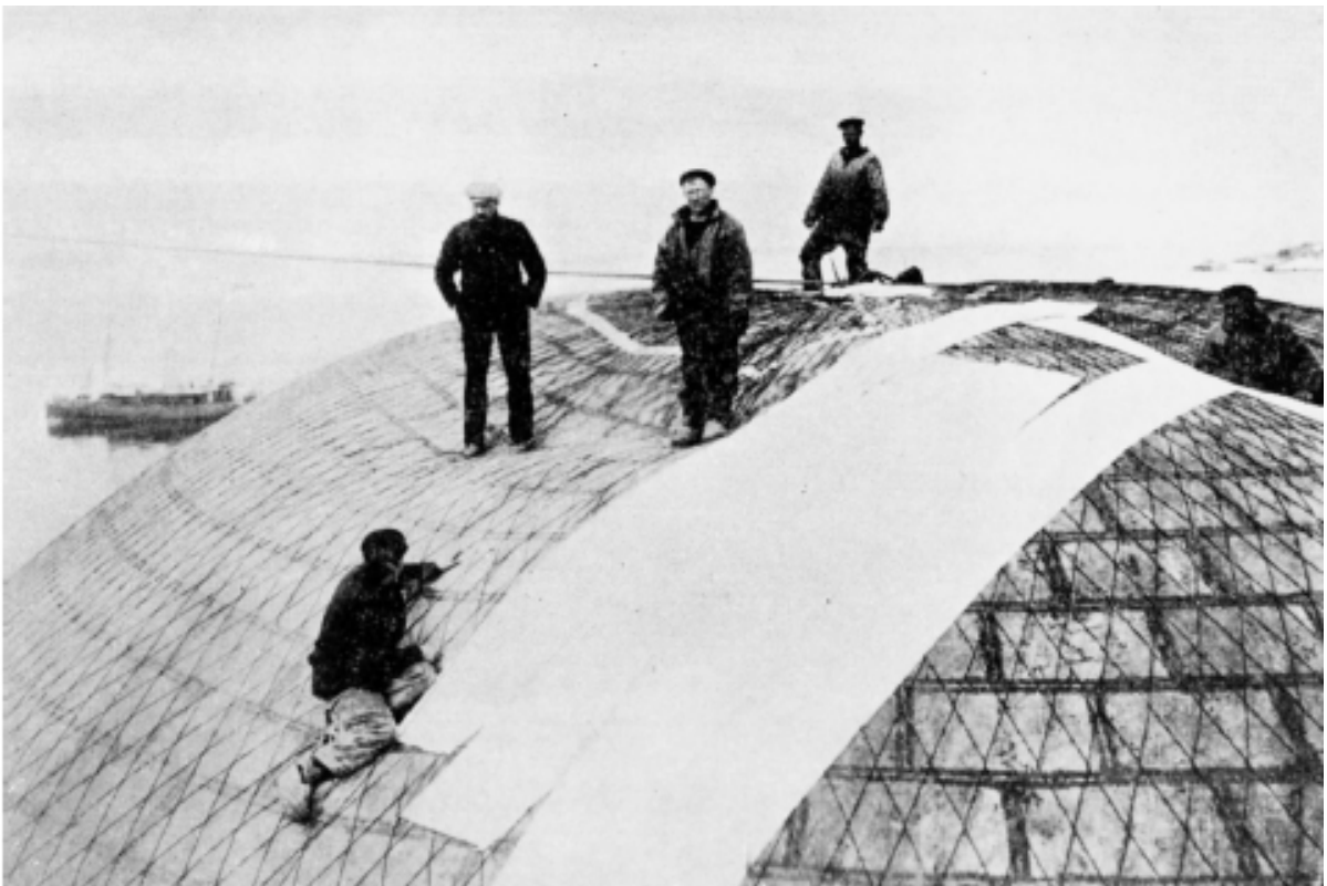
At the base on Dane Island: testing the balloon for leaks.
