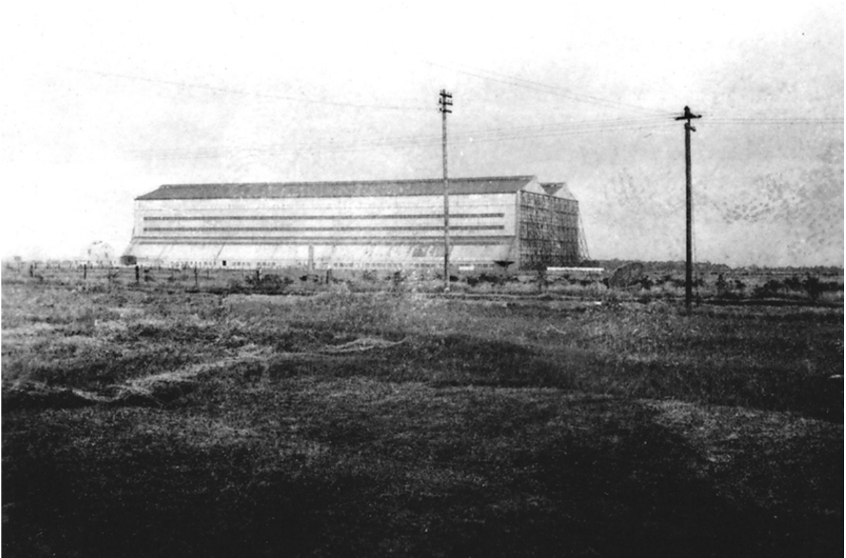
The R100 building shed at Howden, east Yorkshire. (Courtesy Mary Stopes-Roe)
