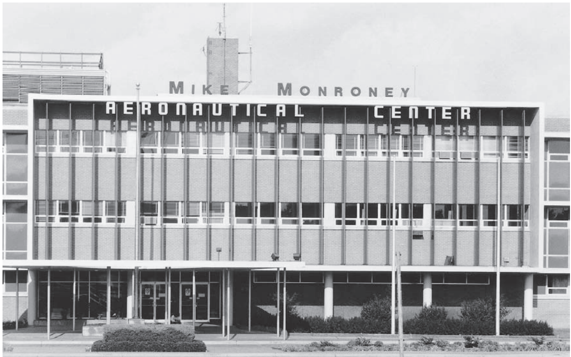
Figure 13–3. The Aeronautical Center Headquarters building in Oklahoma City.
