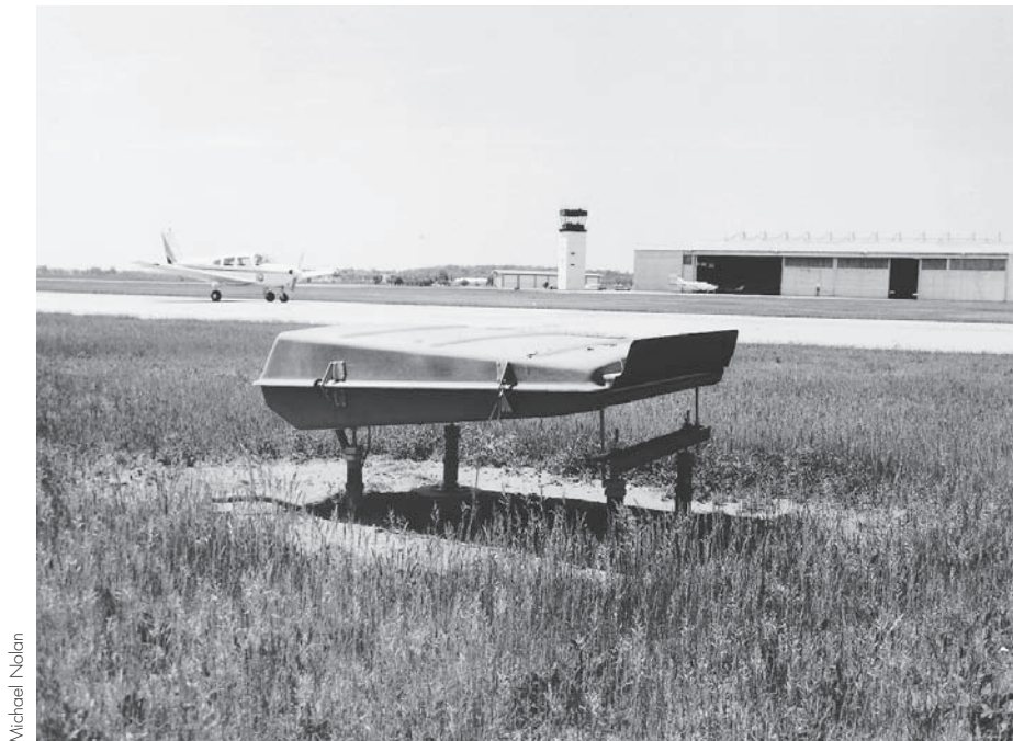
Figure 2–75. A typical VASI light installation.
