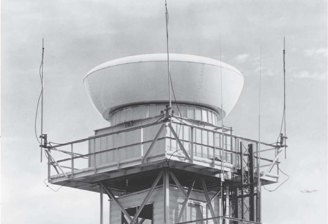
Figure 8–19. Airport surface detection radar antenna and housing.
