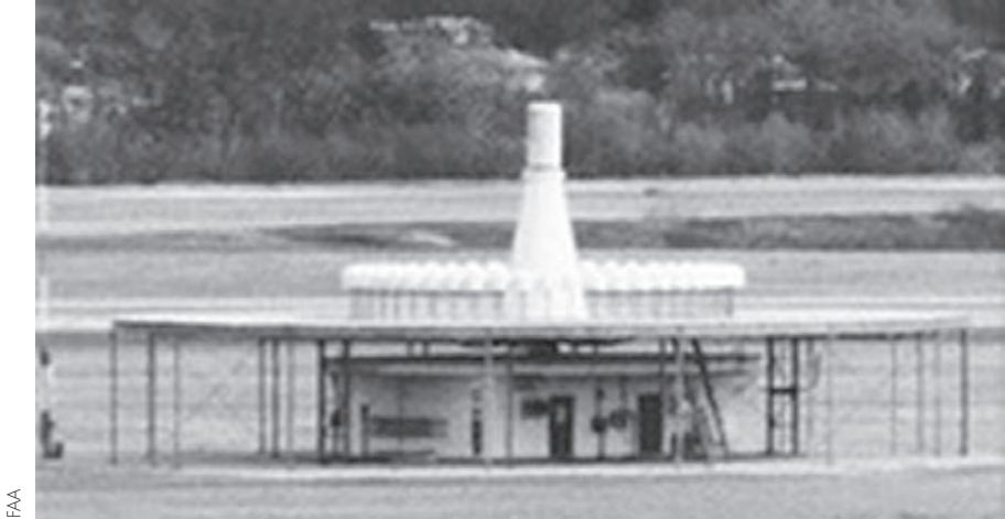
Figure 2–21. A Doppler VOR station.
