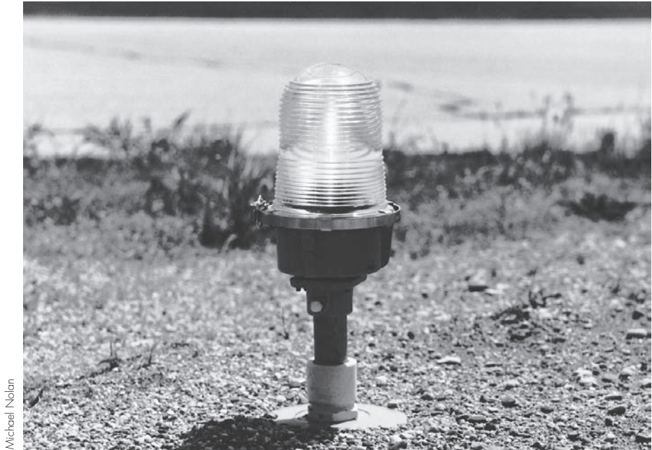
Figure 2–66. A typical runway Fresnel light installation.
