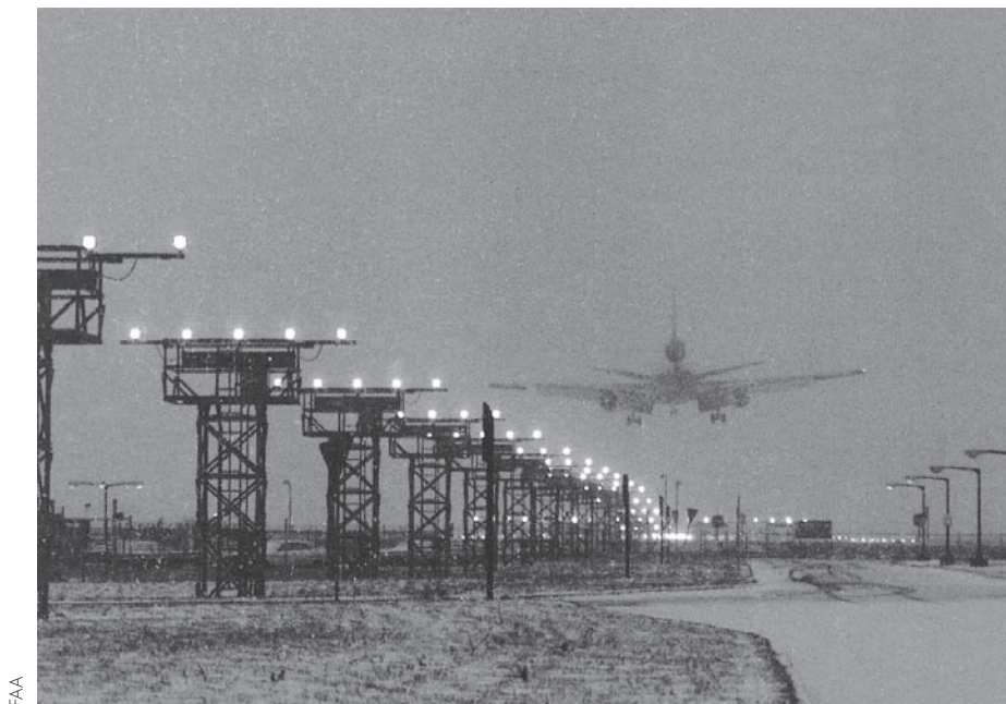
Figure 2-70. High-intensity approach lighting system. (FAA)
