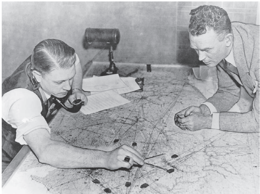
Figure 1–5. Controllers at the Newark ATCU separating en route traffic using maps and shrimp boats.
