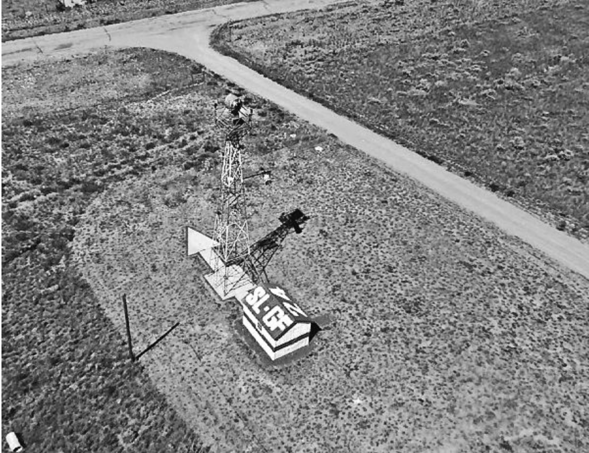
Figure 3: Beacon, steel tower, shed, and concrete directional arrow, beginning Transcontinental Air Mail Route, 1925
