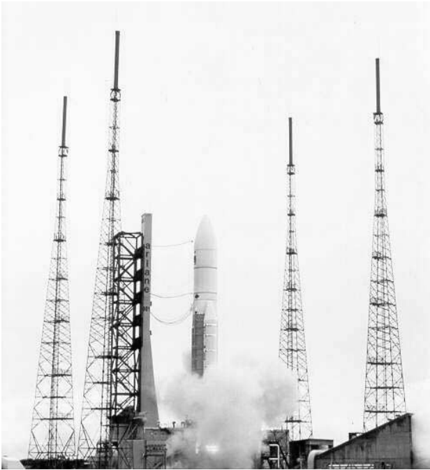
FIGURE 11.9 Lightning protection system on Kourou's ARIANE 5 launching pad (courtesy ESA/CNES).
