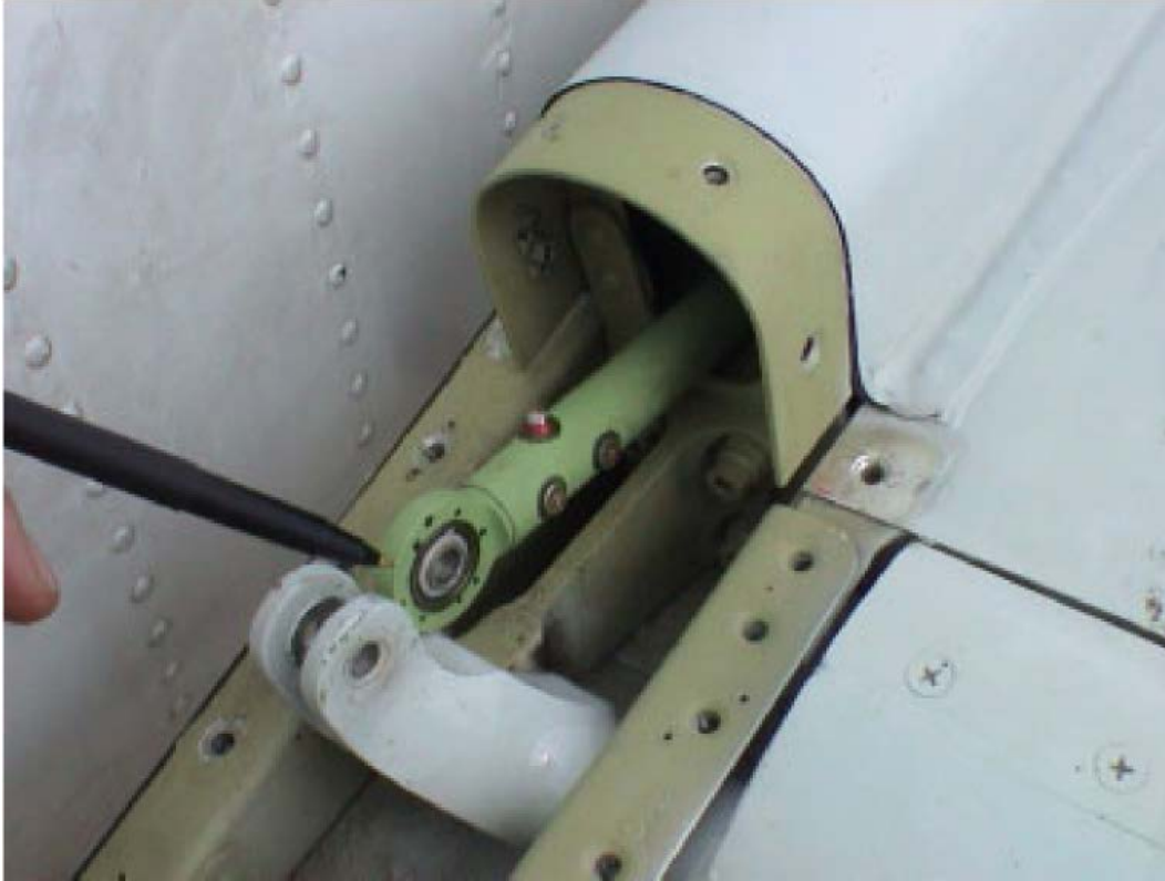
Figure 4.44 Photograph of the Right Elevator Control Tab Pushrod Contacting the Crank Fitting on a Test Airplane (Courtesy NTSB)
