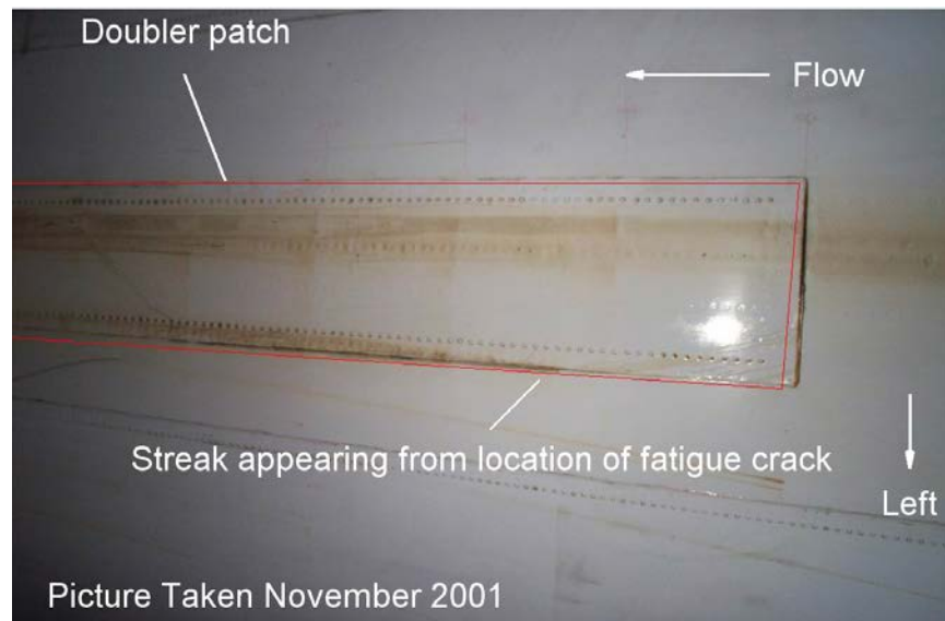
Figure 7.24 Repair Doubler Showing Streaks Emanating from Fatigue Crack (Courtesy Republic of China Aviation Safety Council)
