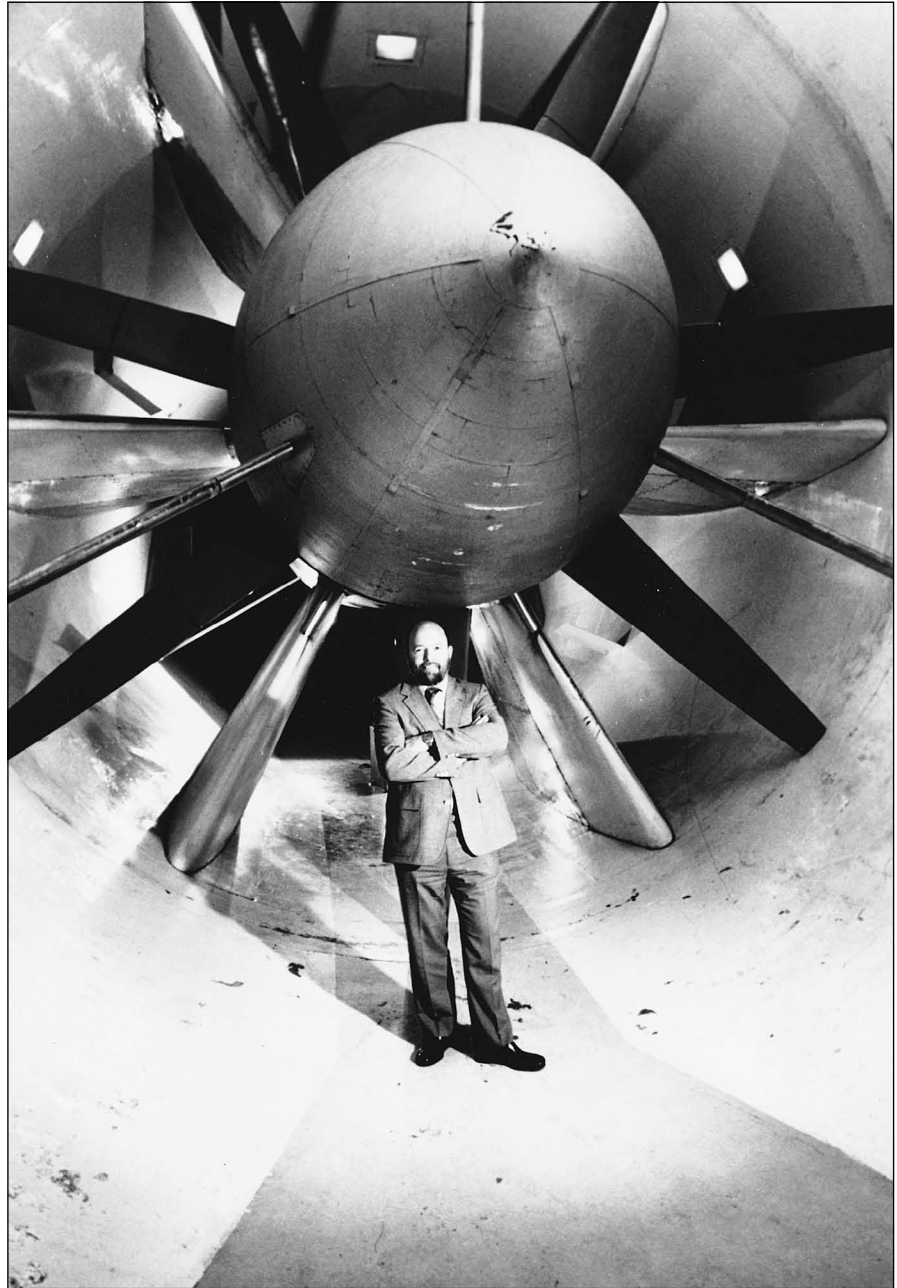
Figure 3.9 (continued) (b) The power fan drive section of the Glenn L. Martin Wind Tunnel. (Courtesy of Dr. Jewel Barlow, University of Maryland.)
